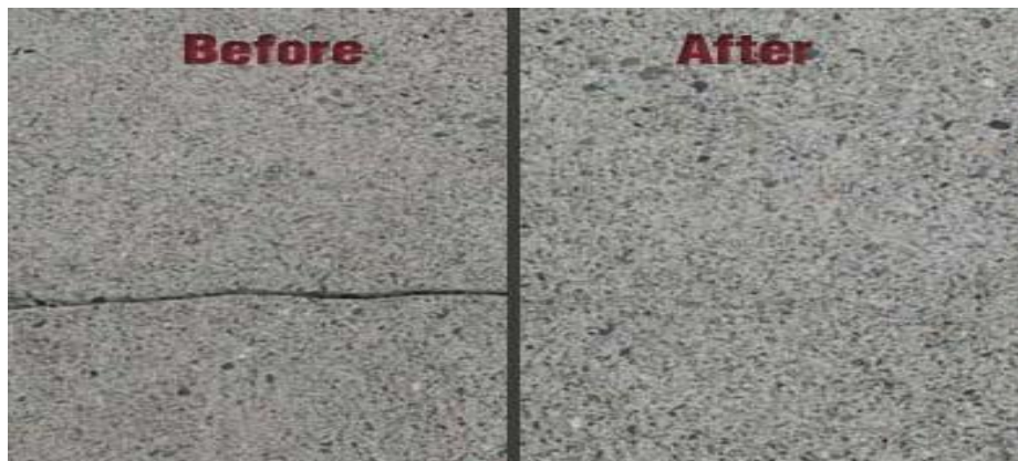
Figure 20: Portland cement grouting (Nojimu, 2007)
