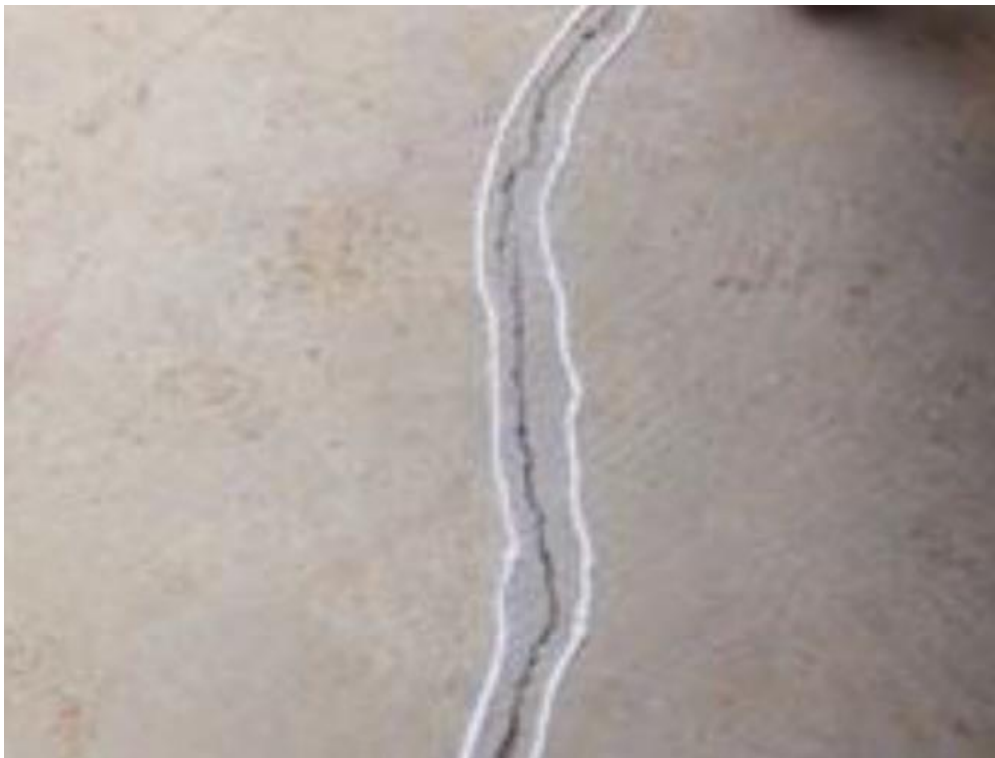
Figure 33: Shrinkage crack repair using dry packing (Sika, 2016)
