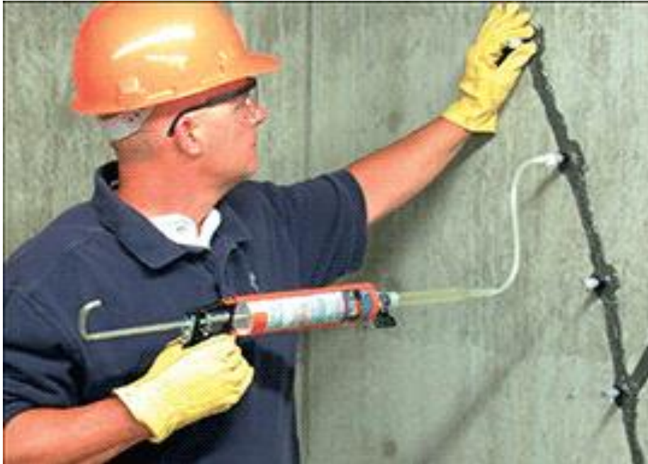
Figure 18: Crack injections using epoxy resins (Nomura, 2013)
