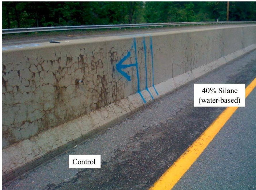
Figure 26: Visual contrast between control section on the left and a section treated with water based saline on the right at Massachusetts site (Michael et.al, 2013)
