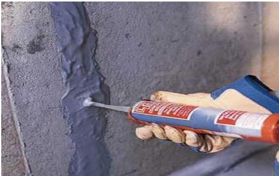
Figure 19: Crack sealing using polyurethane products (Aoyama, 2013)
