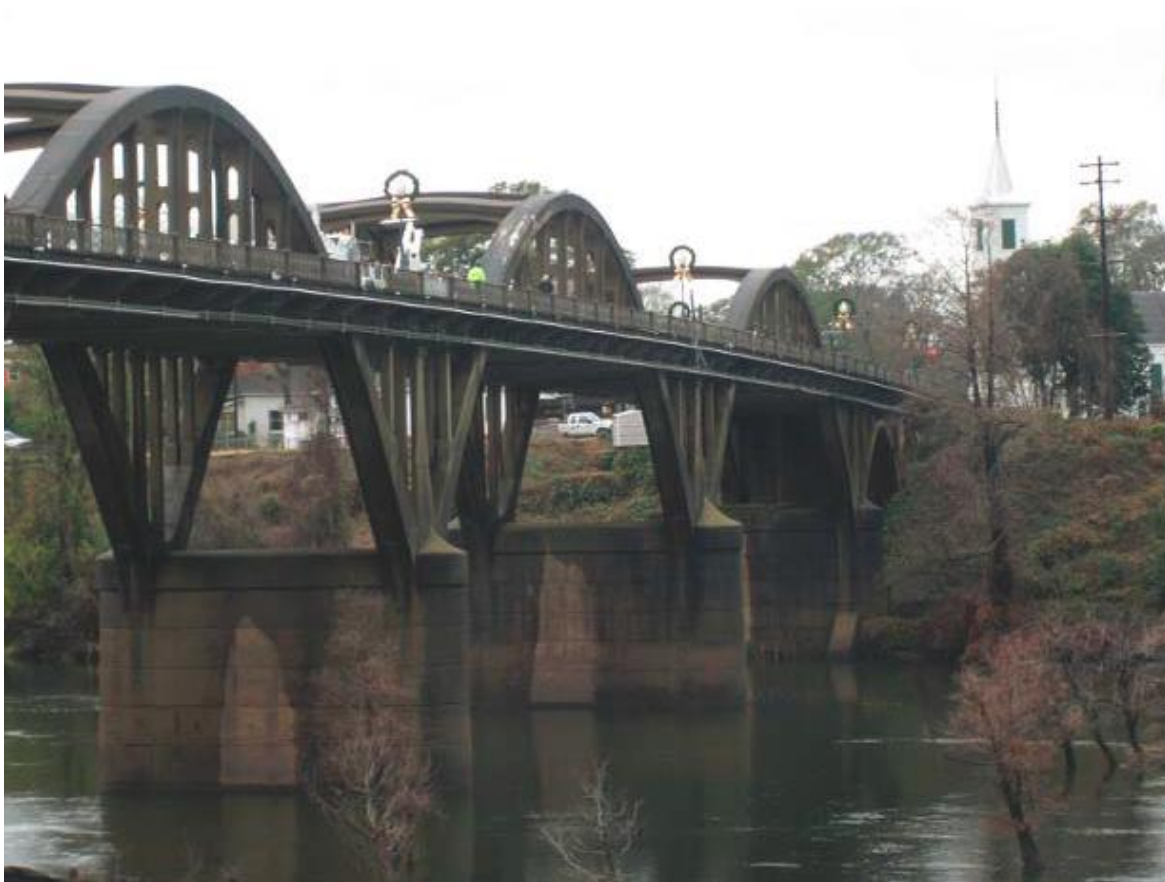
Figure 24: Bibb Grave Bridge north face (Michael et.al, 2013)
