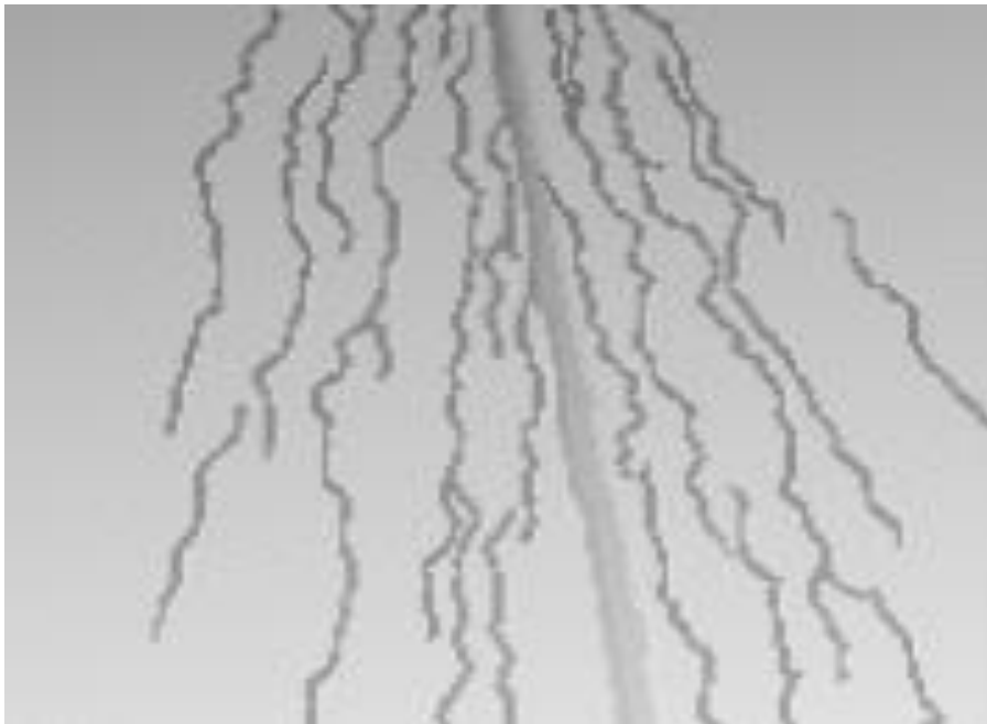
Figure 11: D-cracking near a concrete joint (ACI, 116R)
