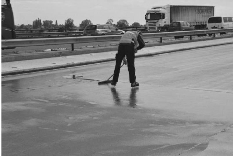
Figure 3-10: Applying the impregnation by hand (Raupach & Büttner, 2014)
