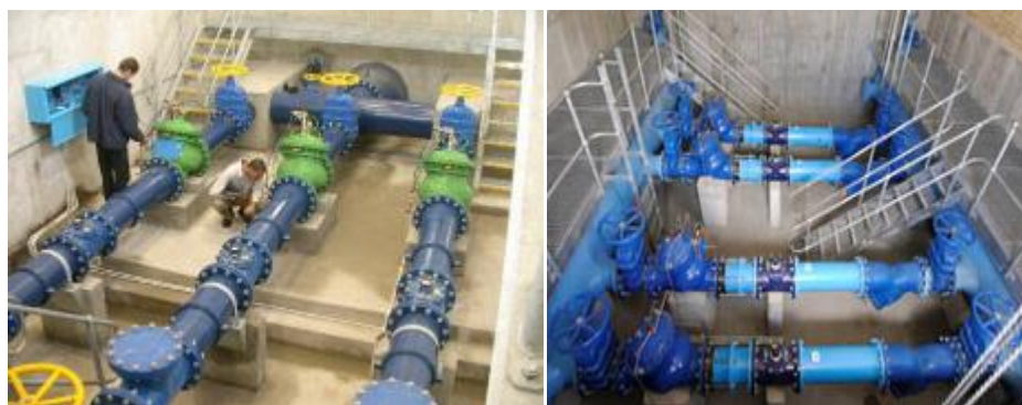
Figure 2.11: Examples of water pressure management system in the City of Cape Town
