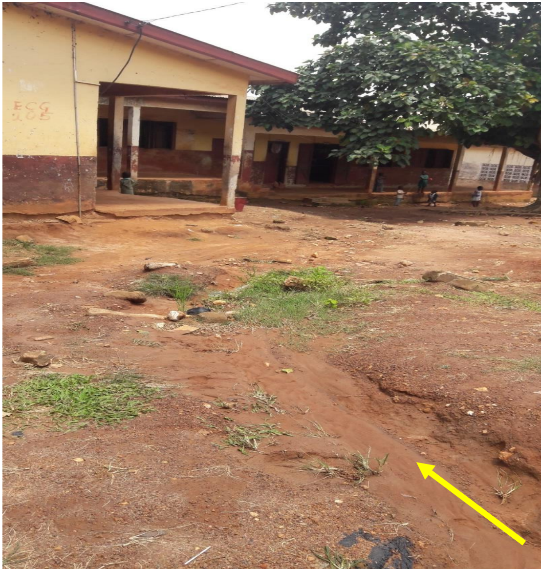
Figure 8 The compound of DBS showing pathways eroded by water
