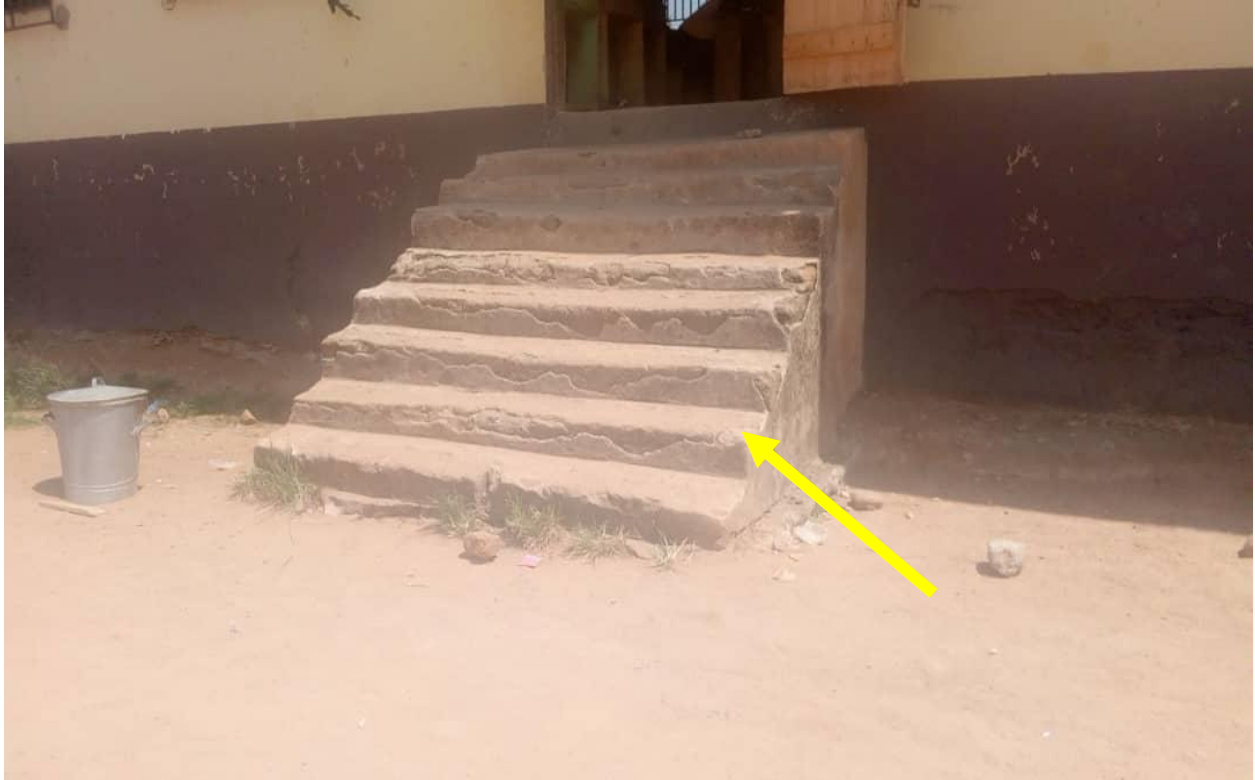
Figure 7 A staircase leading to a classroom in Kamame School Complex
