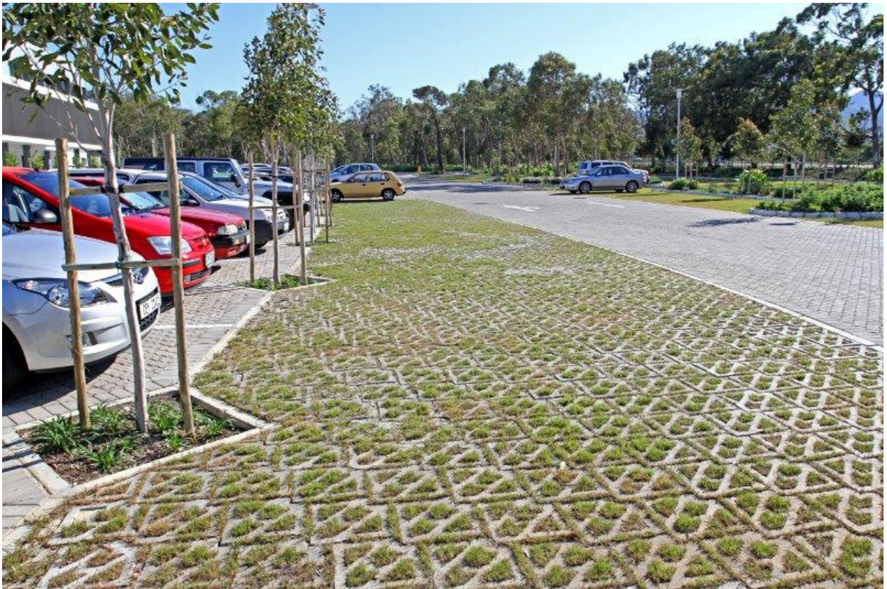
Figure 32, Permeable pavement at Busamed Paardevlei Private Hospital parking area, Strand, Cape Town
