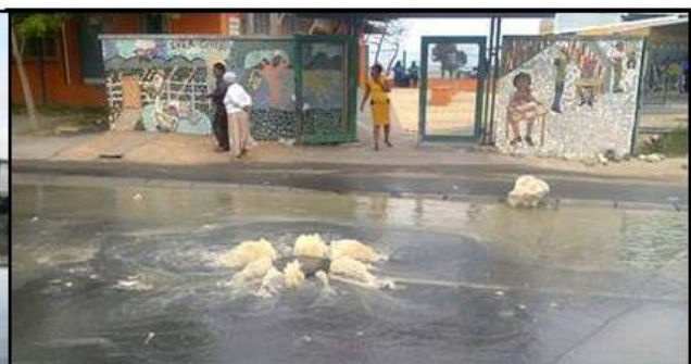
Sewage water from a blocked drain floods the road to the library in Philippi in 2014. Photo by Siphonathi Mbozo Source: http://www.groundup.org.za/article/city-blames-irresponsible-residents-philippi-flooding_2301/
