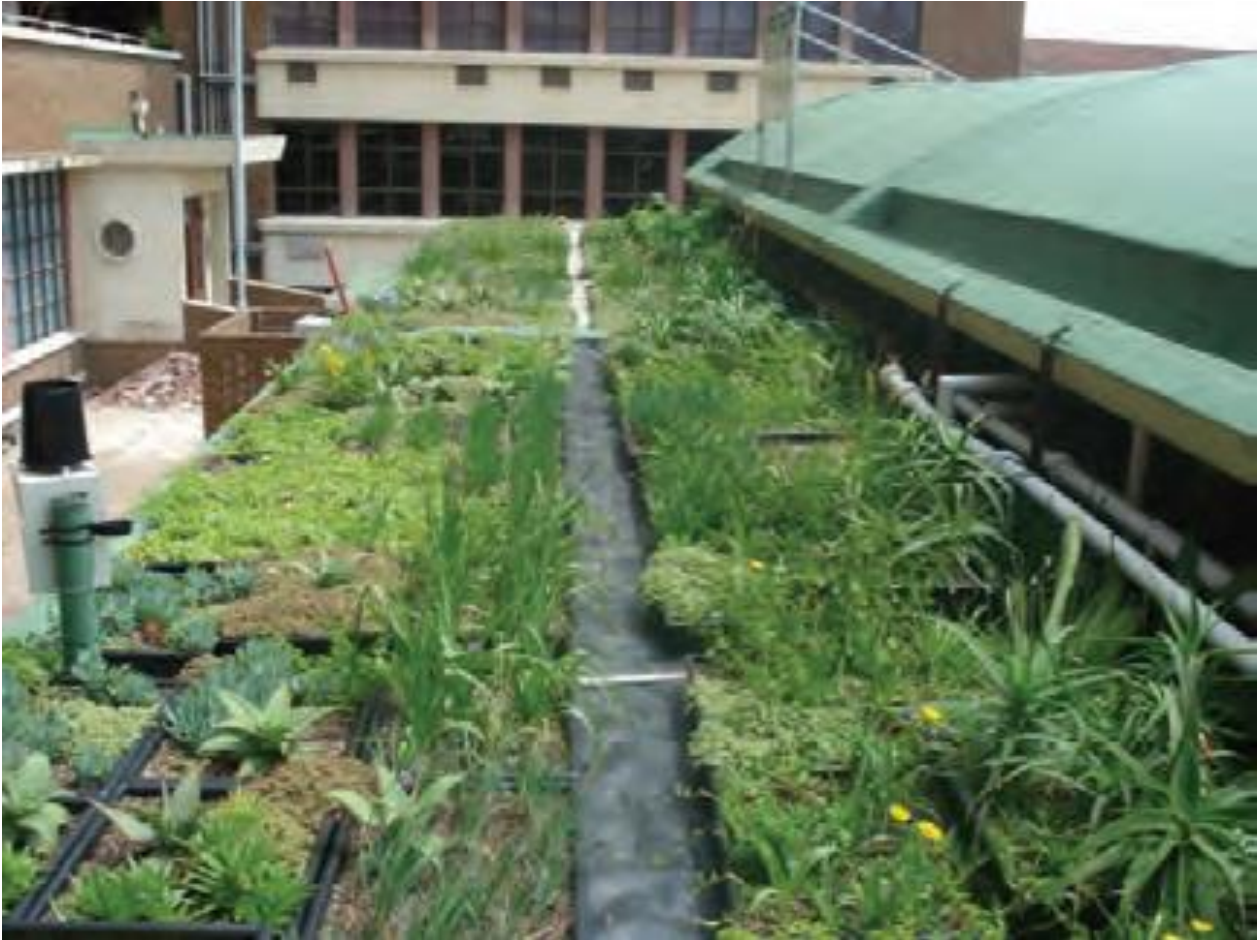
Figure 34, eThekweni Green Roof Pilot Project, Durban CBD (Armitage et al, 2013)
