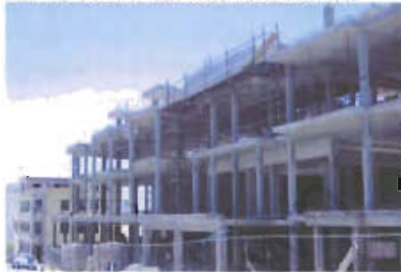
3 New construction at Rose Street and Shortmarket Street.
