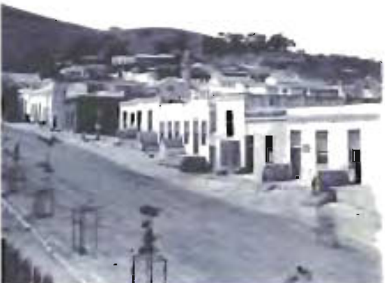
3 periphery Wale Street, looking up towards the Bo-Kaap. Source: CA E-1939
