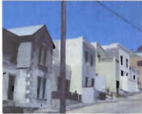
2 Renovations at Shortmarket Street.
