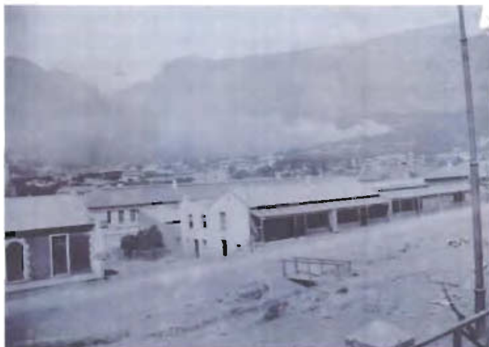
2 Open ditch along Buitengracht Street, demonstrating lack of street improvements. Source: NI.S.A.
