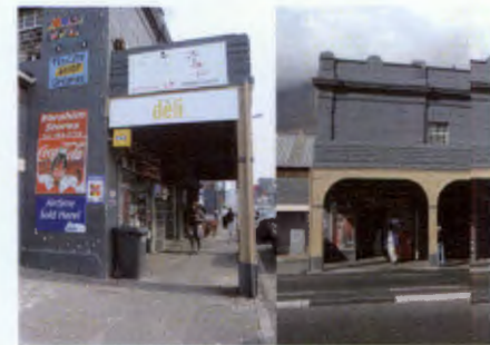
10, 11, 12. Erf 8104 Heritage Building
