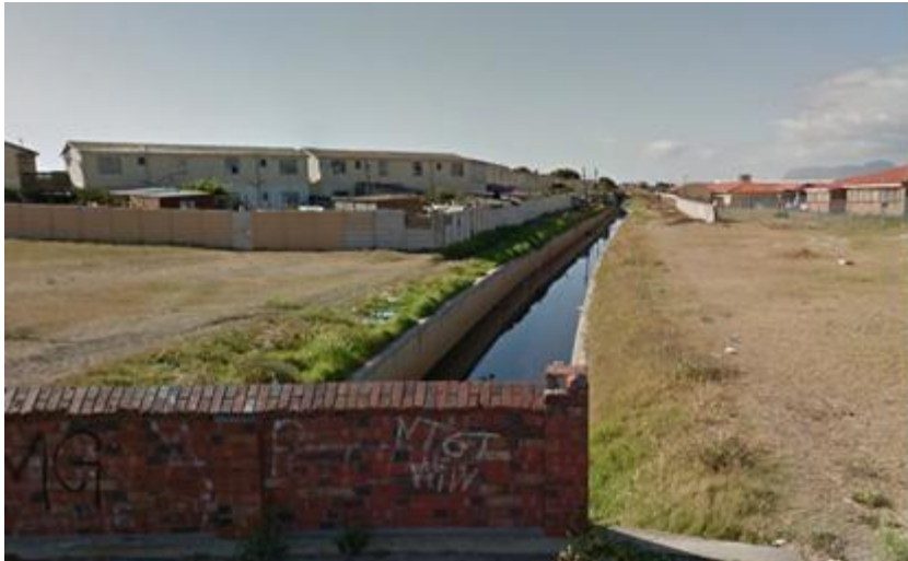
Image 10: MOU on the right, apartment blocks and informal houses on the left.
