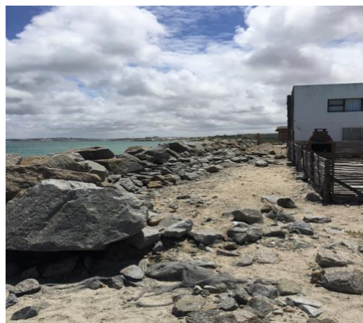
Figure 14: A house which lost its front section due to the 1997 storm (source: author's own)
