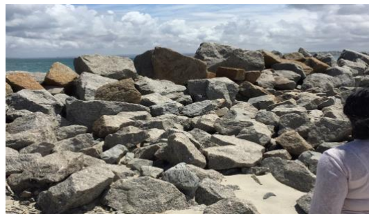
Figure 13: Rock revetments, the emergency response after the 1997 storm (source: author's own)
