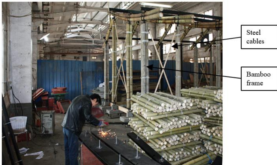
Figure 6.30: Construction and preparation of bamboo culms at Tongji University (Anon., 2010)
