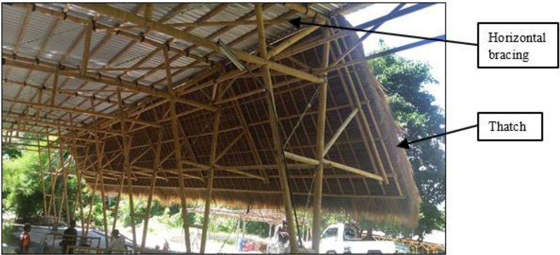
Figure 6.28: Completed warehouse (Cayot, 2016)
