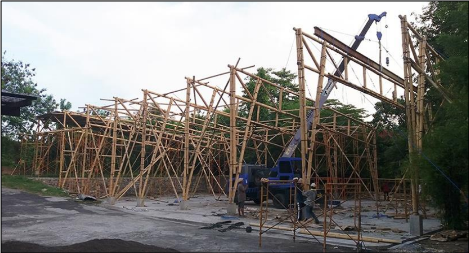
Figure 6.26: Final erection of trusses (Cayot, 2016)
