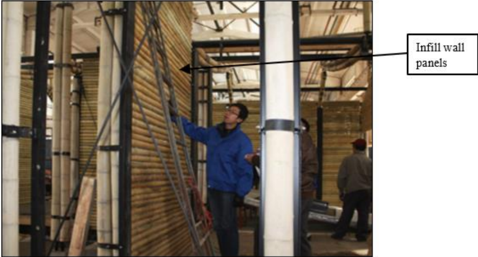
Figure 6.31: Construction of the house at Tongji University (Anon., 2010)
