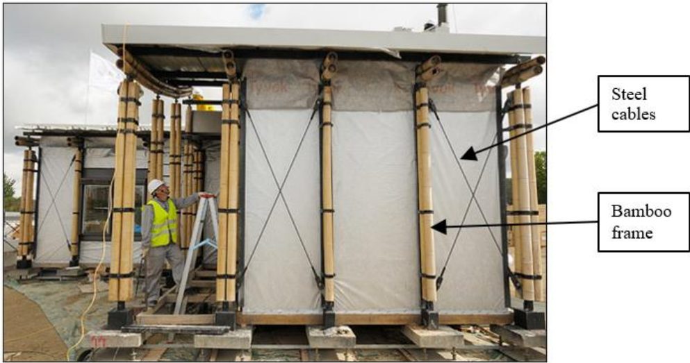
Figure 6.33: Construction phase on site (Anon., 2010)
