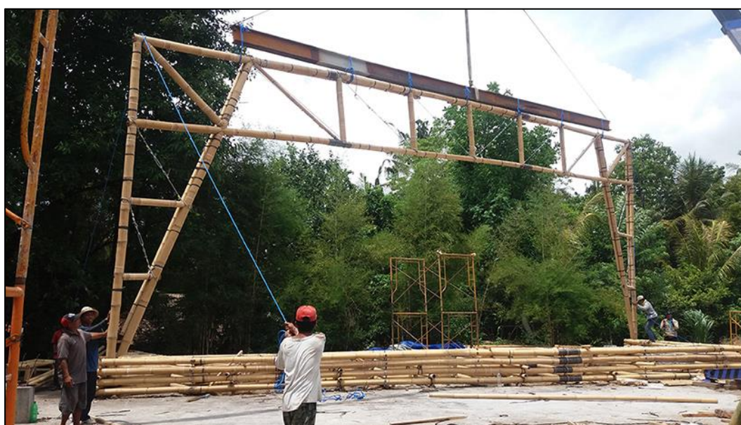
Figure 6.25: Truss erected on site using a 22 m crane (Cayot, 2016)
