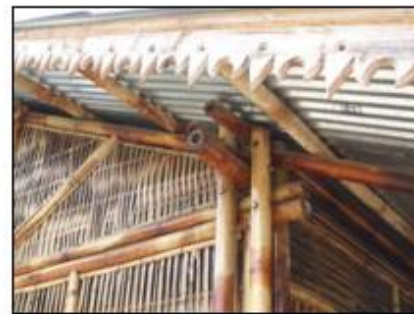
(e) Bolted connection used to connect primary framing
