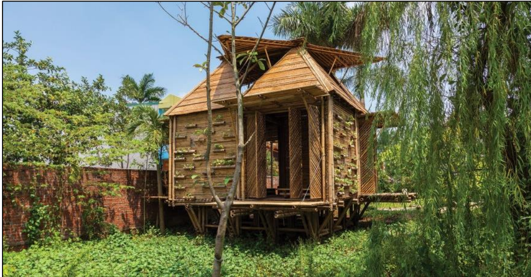
Figure 5.16: Prototype of a bamboo house in Costa Rica with an elevated floor (Berg, 2016)
