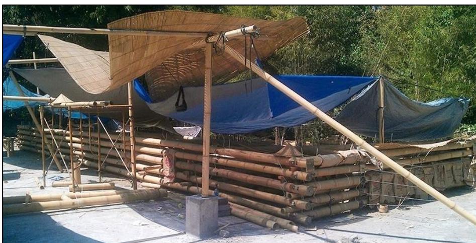
Figure 6.23: Trusses stored on site (Cayot, 2016)
