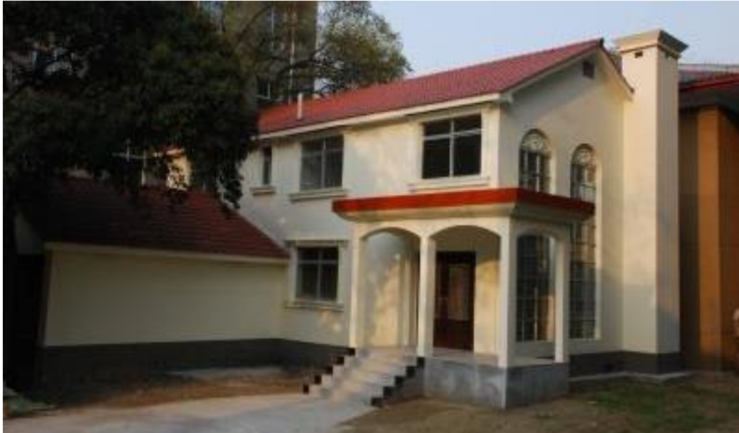
Figure 4.13: GluBam concept house in Changsha, Hunan Province, China, 2009 by researchers at the University of Southern California (Aijazi, 2013)
