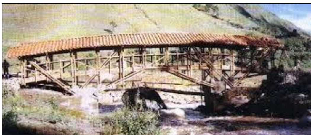
Figure 6.8: Bamboo arch bridge (Stamm, 2004)
