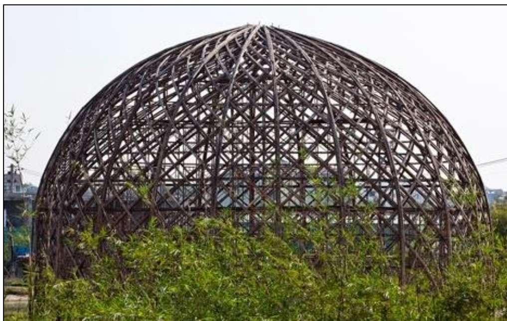
Figure 6.39: Pavilions during construction (Nghia, 2015)
