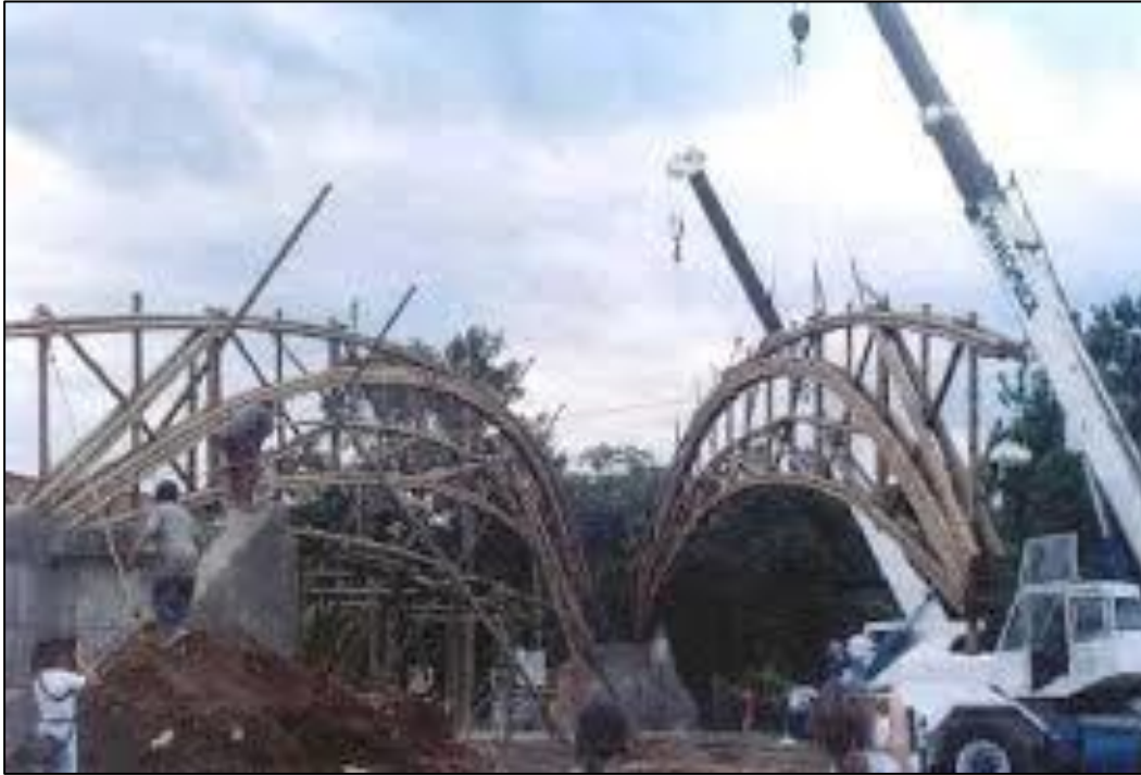
Figure 6.15: Side trusses in place for Pereira bridge (Stamm, 2009)
