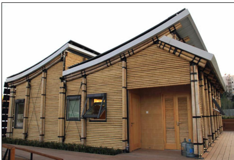
Figure 6.29: Exterior view of the completed house (Anon., 2010)
