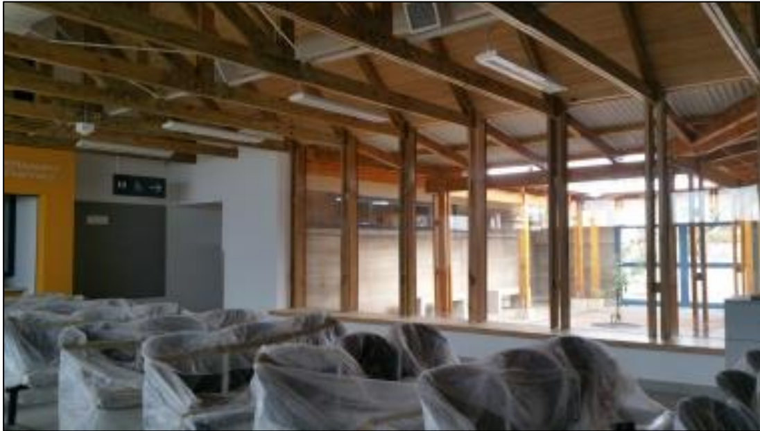
Figure 4.15: Beaufort West Hillside Clinic during construction (WCGTPW, 2018)
