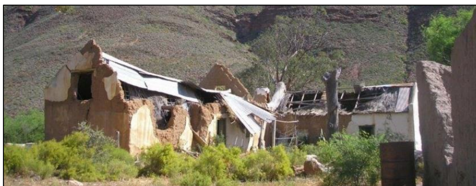
Figure 7.15: Derelict bamboo building outside Vredendal (NBASA, 2017)
