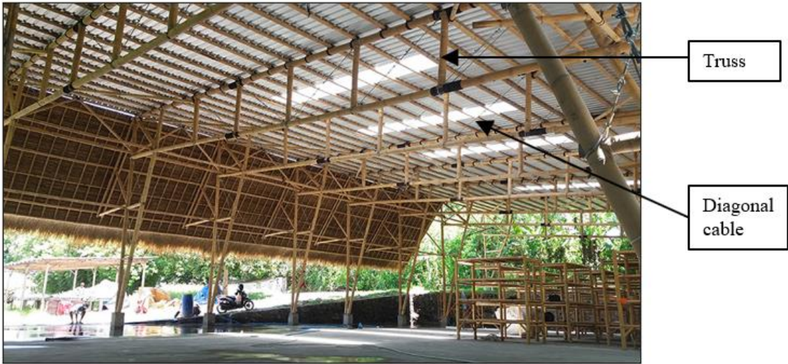
Figure 6.27: Completed warehouse (Cayot, 2016)
