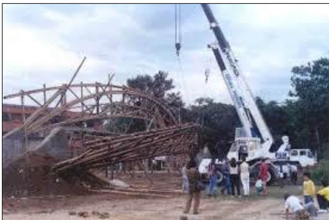
Figure 6.14: Lifting side truss of Pereira bridge (Stamm, 2009)
