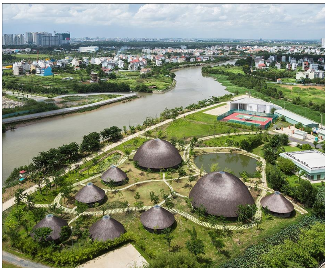
Figure 6.34: Diamond Island Community Centre (Nghia, 2015)
