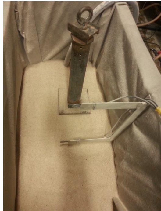
Figure 3-11: Compacting sand at 300mm interval
