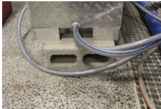
Figure 3-25: Drainage outlets of tank
