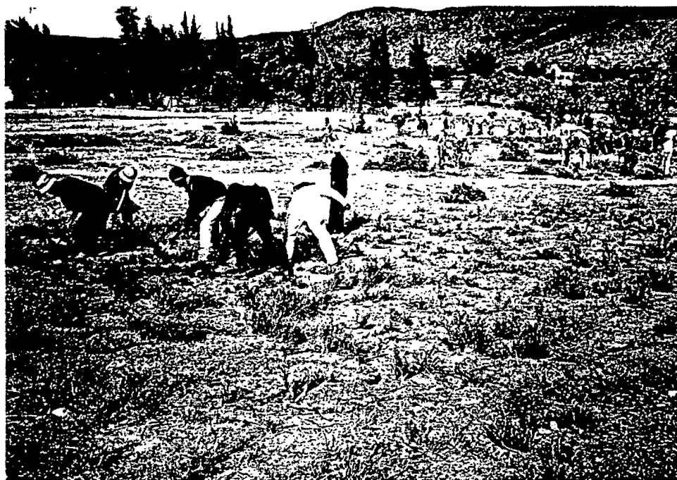
Labourers employed with IDT funds constructing the new soccer field.
