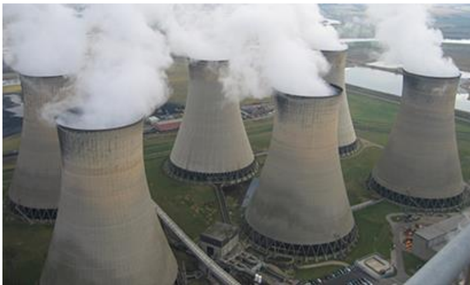
Figure 2-33: Reinforced Concrete Hyperboloidal Cooling Tower Shell Structure( https://www.zenithstructural.com/structural-access-repair-specialists/cooling-towers/,n.d )
