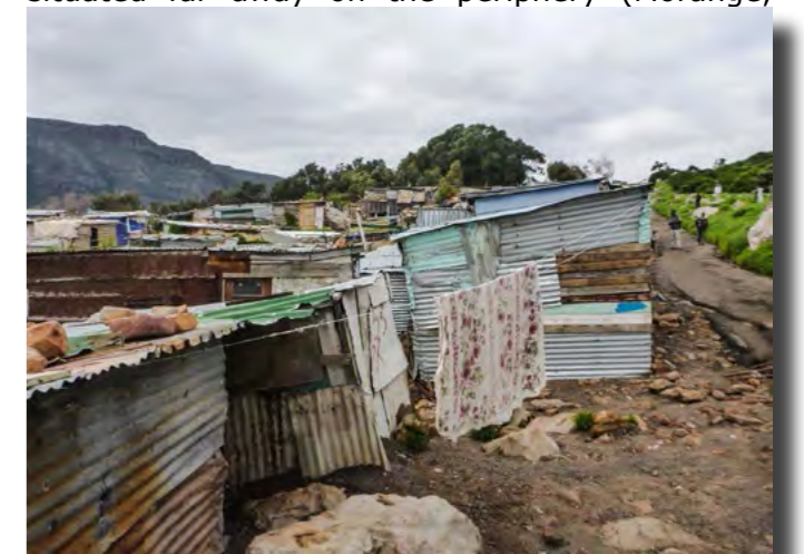
Figure 3.1: Shacks constructed out of flammable, recycled materials
