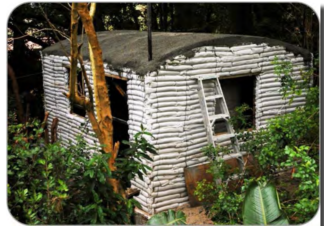
Figure 6.11: The finished structure before the exterior is coated. The design and materials have a much higher fire resistance ( http://e-khaya.com/ , 2013)
