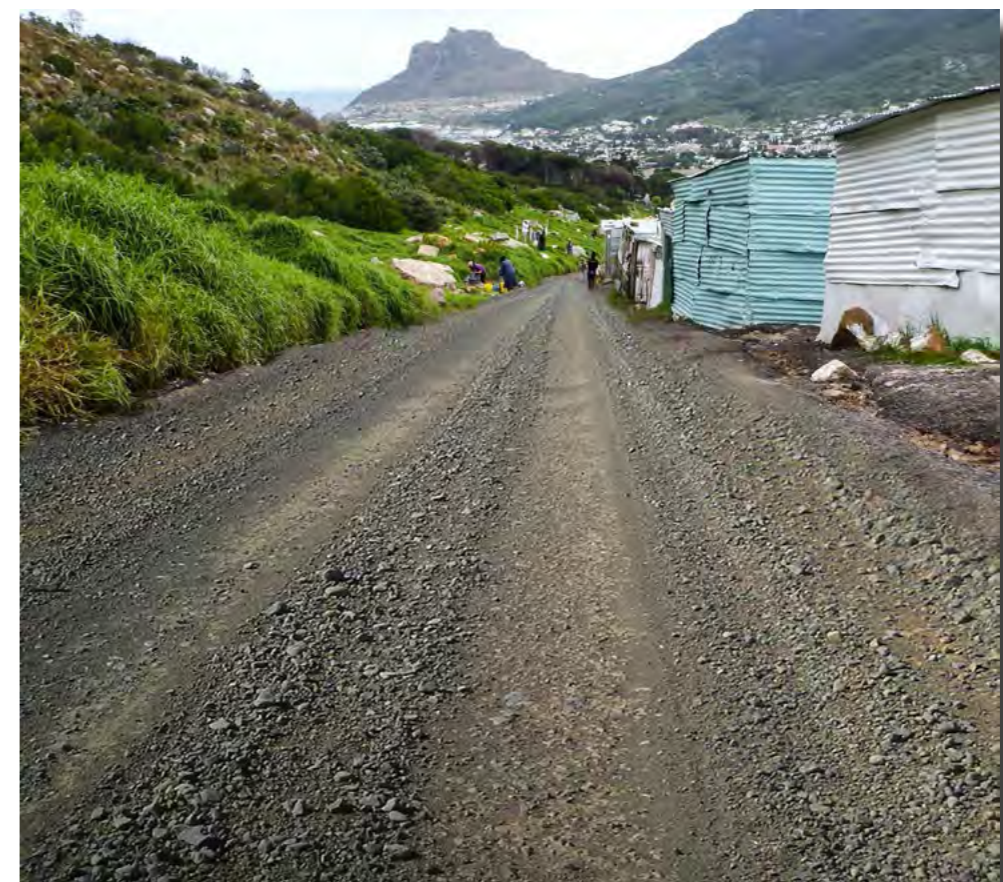
Figure 6.14: Improved Road surface; smooth, less steep, accessible (edited Photograph)
