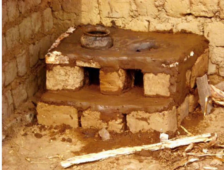
Photo 30: Improved (Army stove) wood burning stove under construction
