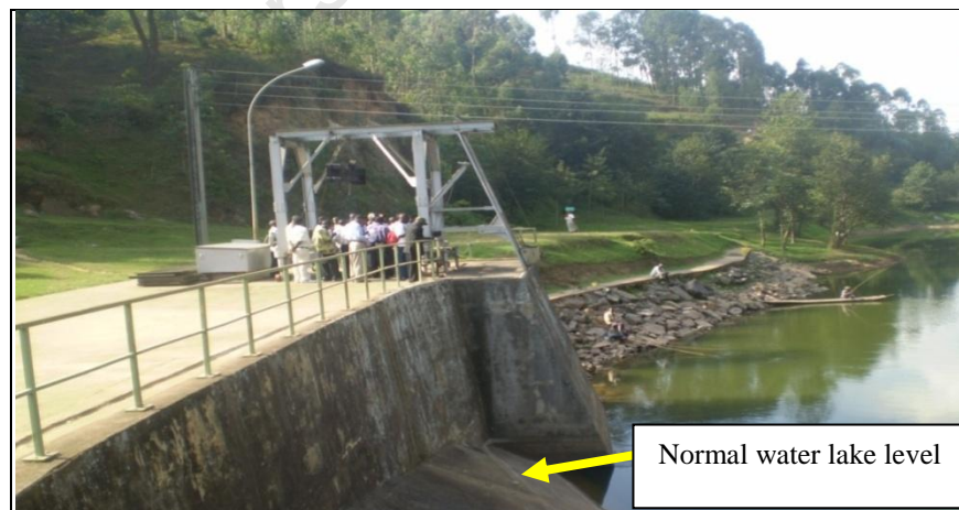
Photo 3: Water level Lowering at Mukungwa hydropower catchment (2008)
