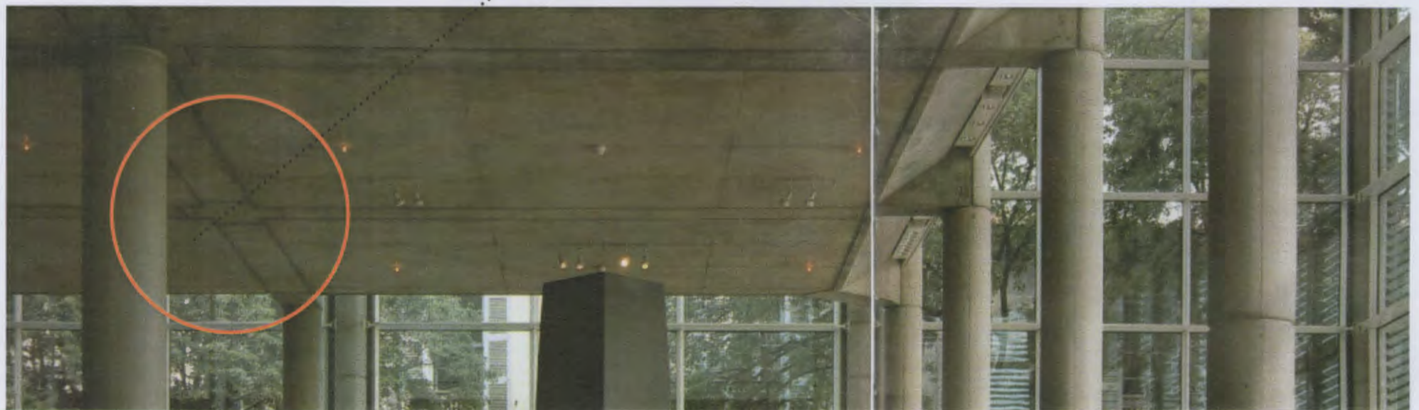
Columns, up-stand beams and floors bevelled up at end of floor plate (January & Roux, 1993, p22 - 23)
