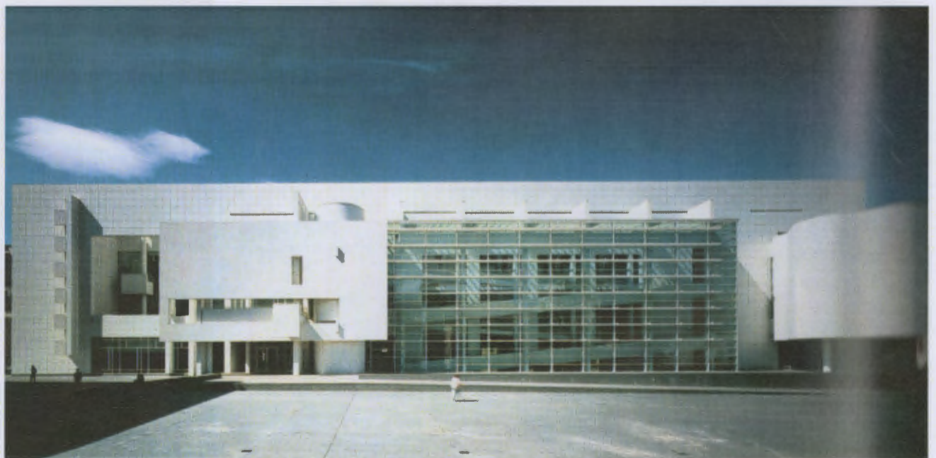
View of the façade from Placa dels Angels – showing the façade as one complex element, despite the building behind being, in effect, two separate buildings (Frampton, 2003, p252)
