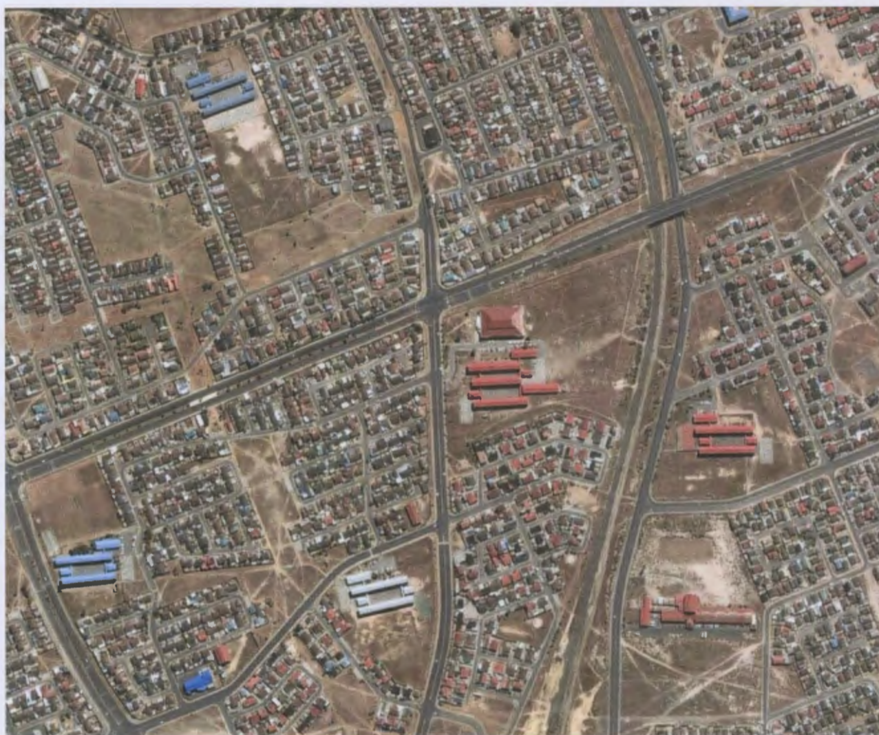
Mitchells Plain - showing identical schools built according to standard plans, most of them without halls, outdoor play areas or sports fields. (Google Earth, 2009) The schools sit in the middle of a large plot of land, surrounded by a fence, make no contribution to a positive public environment and present themselves as introverted.
