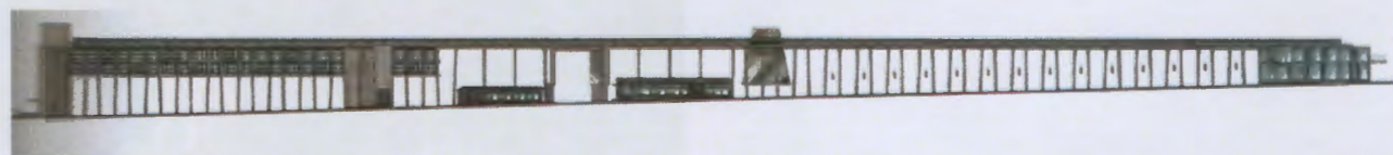
South Structure from Union Road
