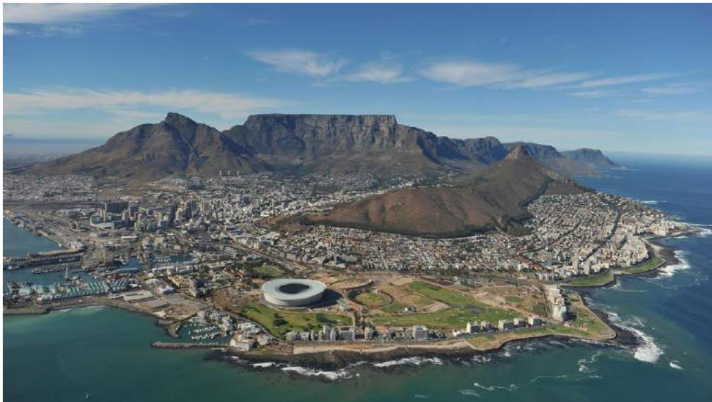
Figure 4 Aerial image showing Cape Town Stadium's context
