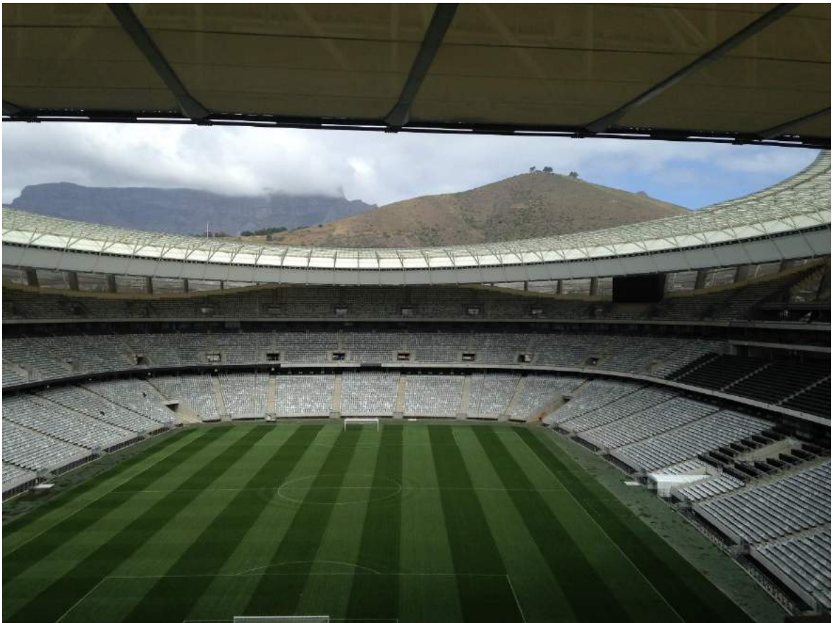
View to the pitch taken from the North side of Level 7
