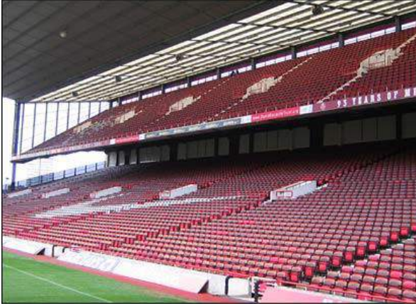
Figure 52 Highbury Stadium before adaptation
