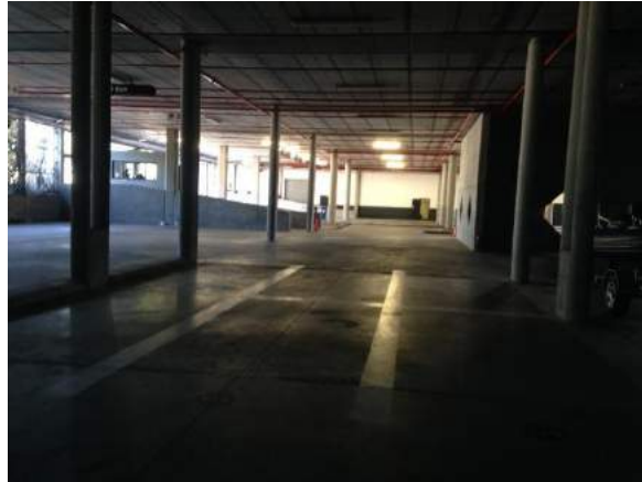
Photograph showing the space of the northern parking area of Level 0
