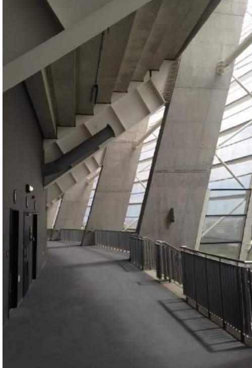
Exposed concrete and steel structure
