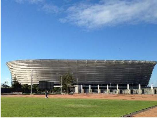
Figure 31 Daytime view of the Stadium showing the facade as opaque
