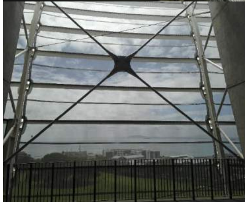
Large views through the fabric façade
