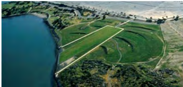
Figure 73: The topography of Candlestick Point Park expresses the dune formations of the land before development, as well as provides sheltered areas in the new park.
