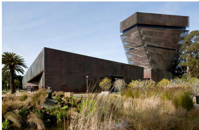
Figure 46: The de Young Museum uses copper panels over its entire facade which have discoloured over time, merging it into the park landscape
