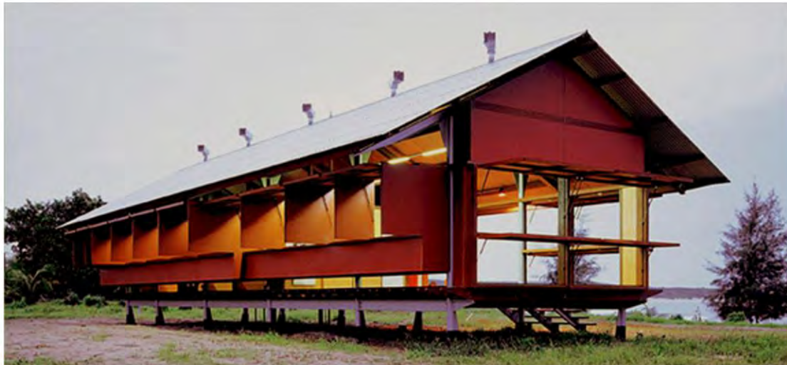
Figure 58: Operable plywood panels allow for flexibility in the permeability of the building envelope, blurring boundaries between nature and building
