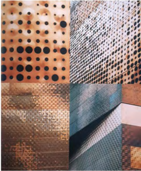
Figure 62: The use of the same material over the entire facade is made more dynamic through the individually patterned and indented panels
