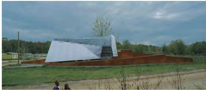
Figure 45: Mason's Bend Community Centre serves as a landmark in its rural landscape, utilising a limited palette of materials which emanate the surrounding natural elements
