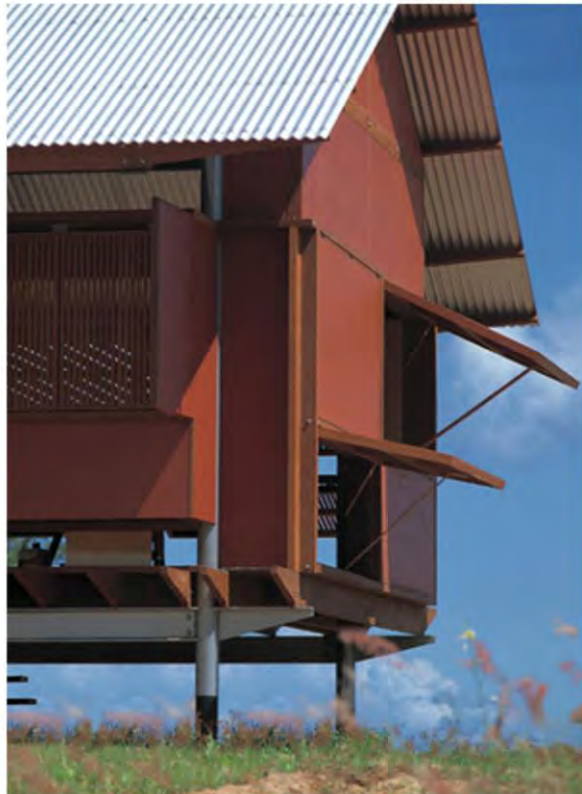
Figure 50: Glazing is rendered unnecessary as operable plywood screens protect the internal space and can be opened up as necessary to provide natural ventilation
