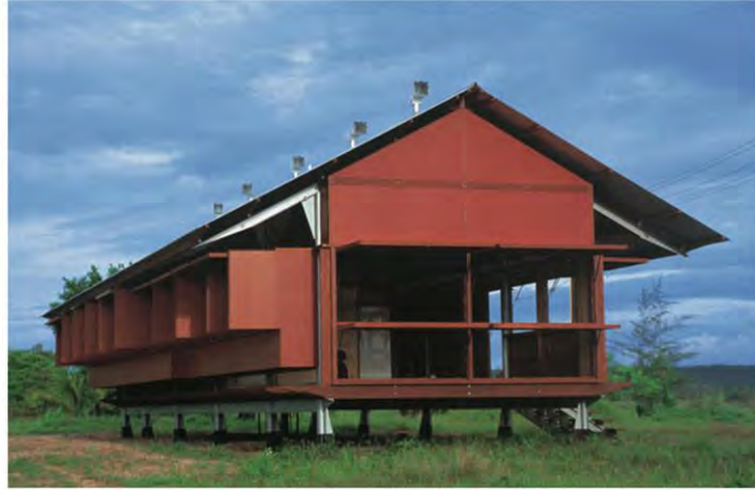
Figure 44: The Marika-Alderton House by Glenn Murcutt - an architectural prototype conceived to respond to the natural landscape and extreme cyclone conditions
