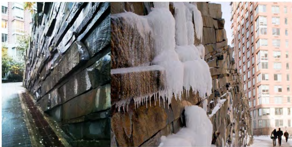
Figure 76: Van Valkenburg's wall at Teardrop Park, Manhattan, is an intervention which relies on the qualities of water to demonstrate the intangible concept of natural process. The noticeable change of the wall at a human scale makes observers aware of changing seasons.
