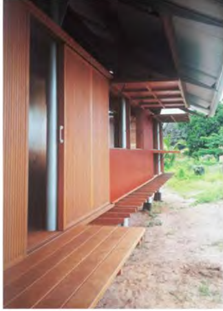
Figure 55: Slatted timber screens provide security whilst still allowing fresh air into the space
