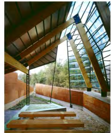
Figure 54: The lighter secondary structure which supports the glazing allows more natural light to penetrate the space
