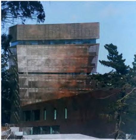
Figure 64: The colour and patterns of the copper panels mimic colours and patterns of the surrounding landscape
