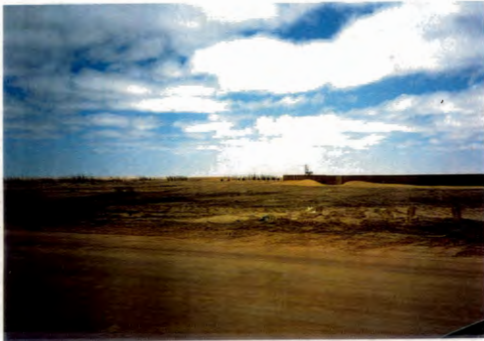
Plate 17b: The town's boundary. The reeds and wall create an edge with the desert. Note how the wall prevents sand from entering into the settlement.
