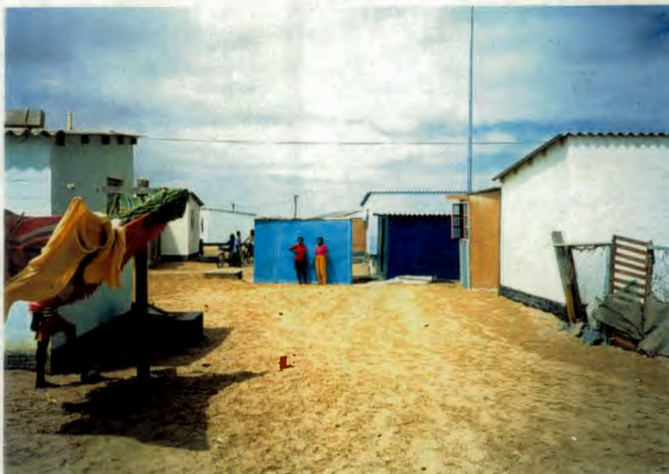
Plate 9: Informal dwelling units in Kuisebmond.
