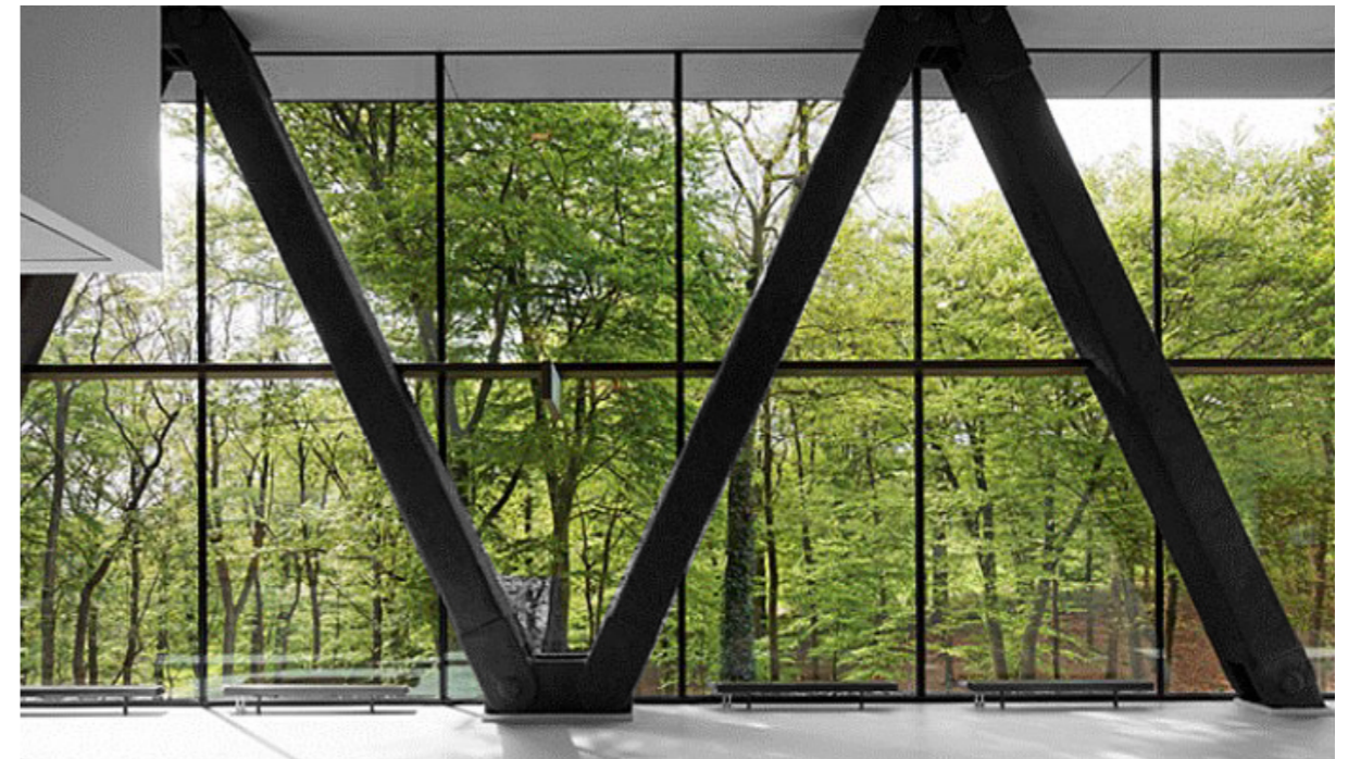
Figure 2.7: View of exterior from internal circulation. Koen van Velsen. Netherlands. 2011
