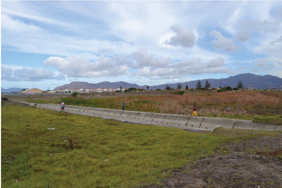
Figure 27 (bottom): Site photograph showing storm water pipe entering the Lotus river from Ottery light industria - looking west.
