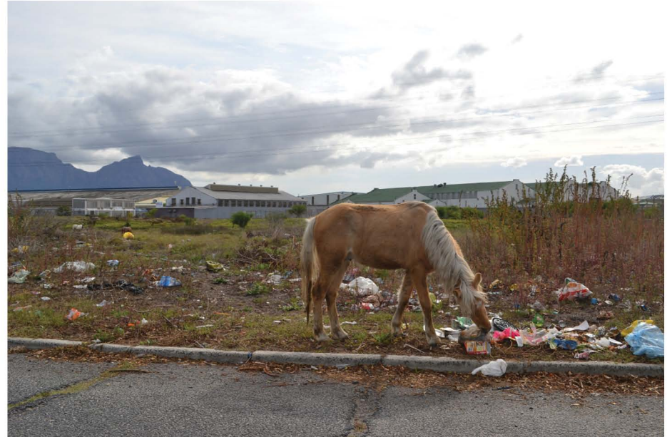
Figure 29 (bottom): Site photograph showing miscellaneous rubbish blocking the canal.
