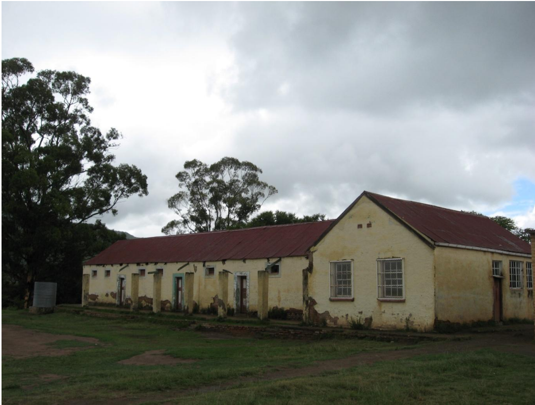
Figure 48 Tamboekiesvlei School, 2011 (Photograph: S I Blackbeard)
