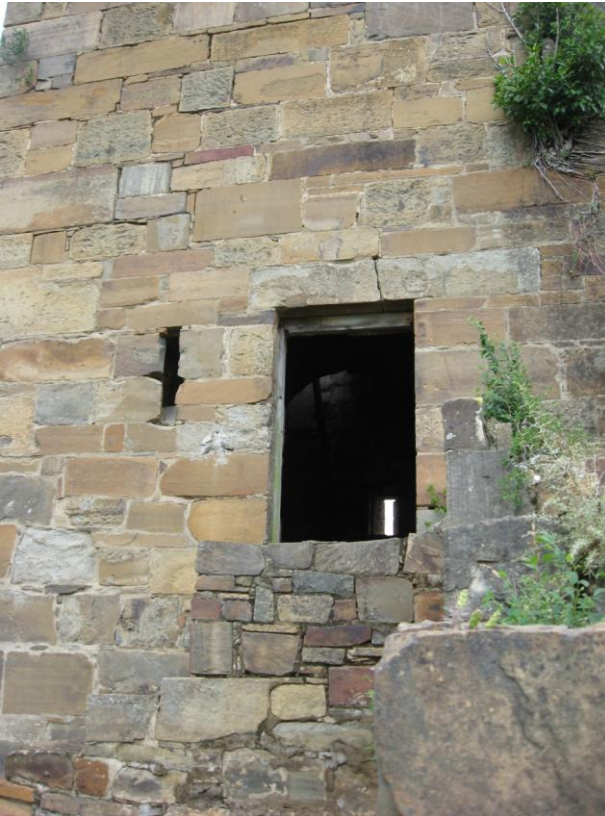
Figure 23 The tower door. 2011 (Photograph: S I Blackbeard)
