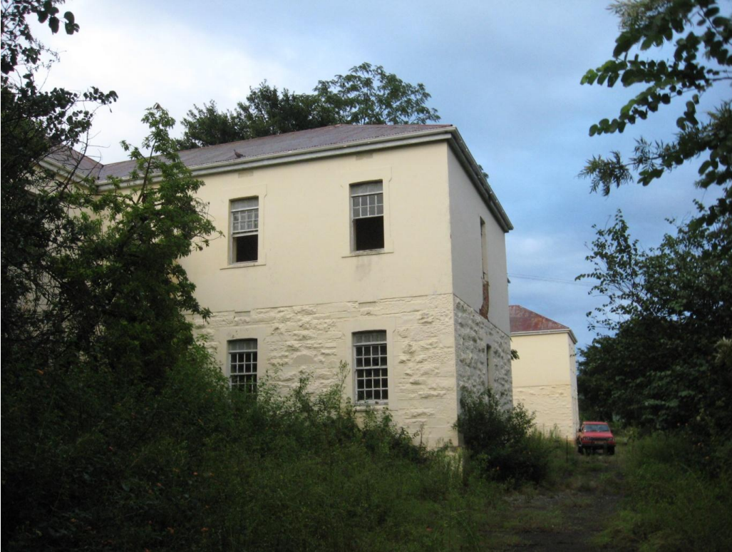
Figure 16 The Fort Beaufort barracks, 2012 (Photograph: S I Blackbeard)
