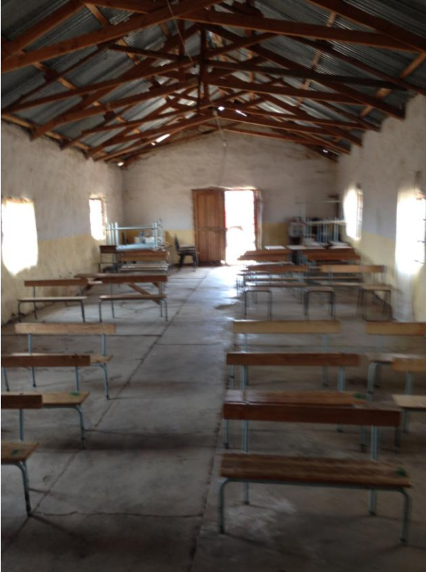
Figure 53 Tamboekiesvlei community hall, 2014 (Photograph: S I Blackbeard)
