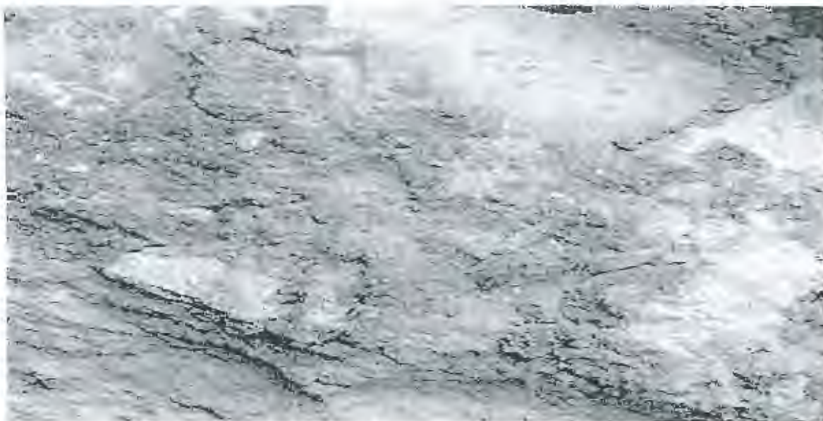
Figure 4.4 Rough surface texture of RCA particle (concrete)
