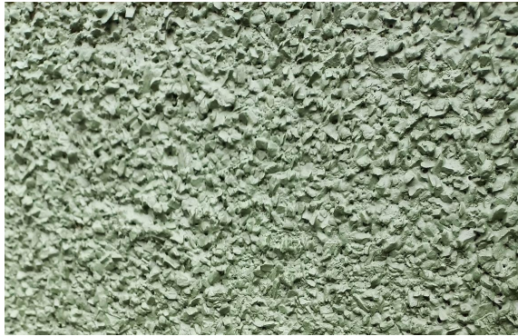
Figure 17. Auwal Mosque front wall texture
