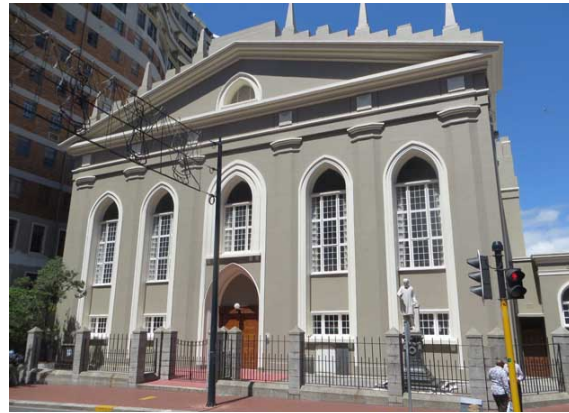
Figure 3. Northwest elevation of Grootte Kerk
