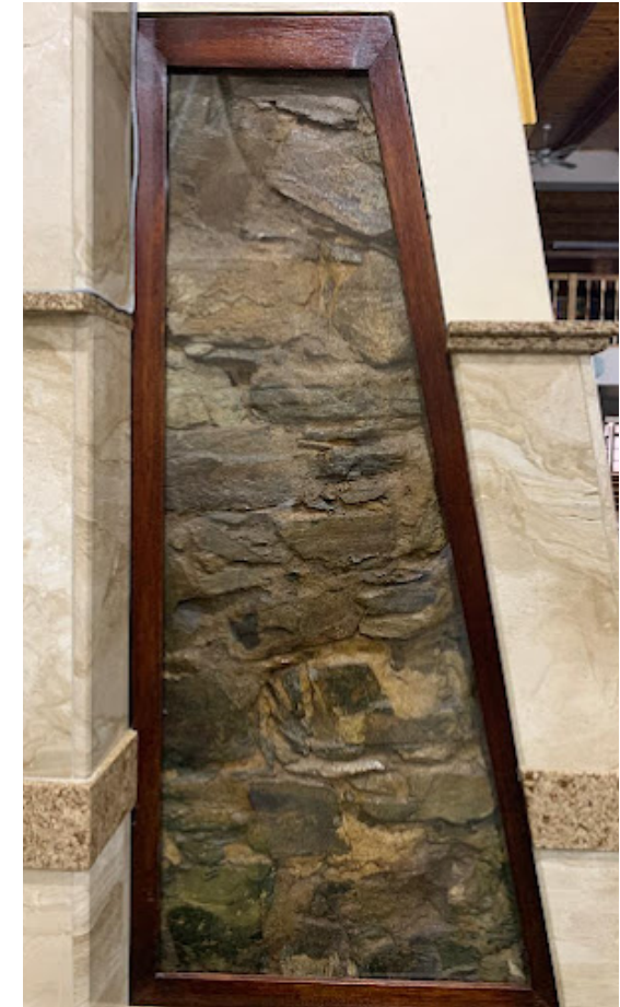
Figure 19. Framed portion of the column's stone structure at Auwal Mosque
