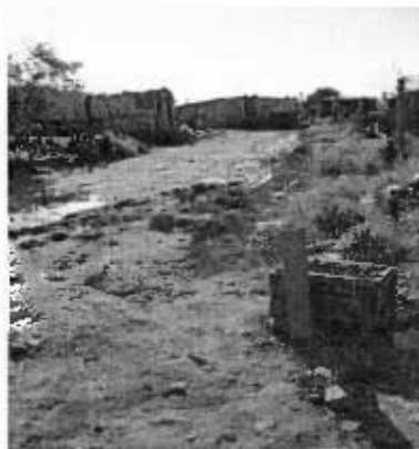
Fig 2: Low Quality (SOS)-Low Standard (LOS): A standpipe with undesirable greywater conditions
