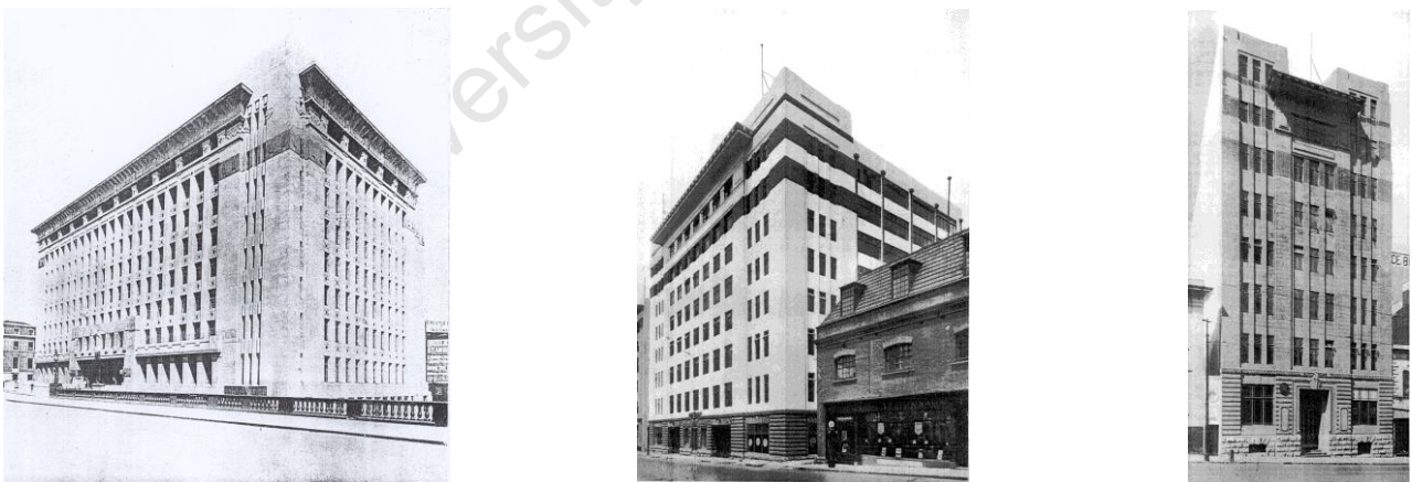
Figure 5: Adelaide House, London, by John Burnet and Boston House by WH Grant (AB&E Oct. 1930)
