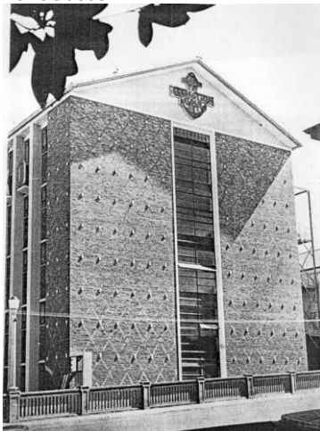
Plywoods offices Parow
