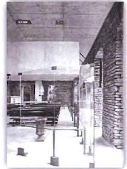
Figure 9a – The walls of the ruin are retained and celebrated on the interior. Simple, unfinished new materials highlight the texture of the old: Chapel, Paulo Mendes da Rocha (Finotti, n.d.)
