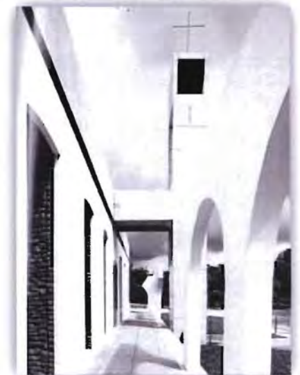
Figure 9b – Ruin walls are plastered on outside and made to look like part of the new: Chapel, Paulo Mendes da Rocha (Finotti, n.d.)
