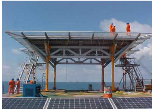
Fig 1.1: Aluminum Helli deck under Construction on Off Shore Facility {28}
