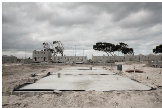
Foundations, Strandfontein Road
