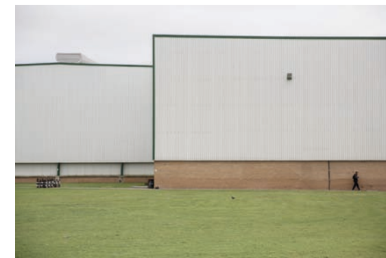
Warehouse, Ottery Road
