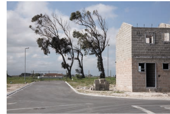
New housing development, Strandfontein Road
