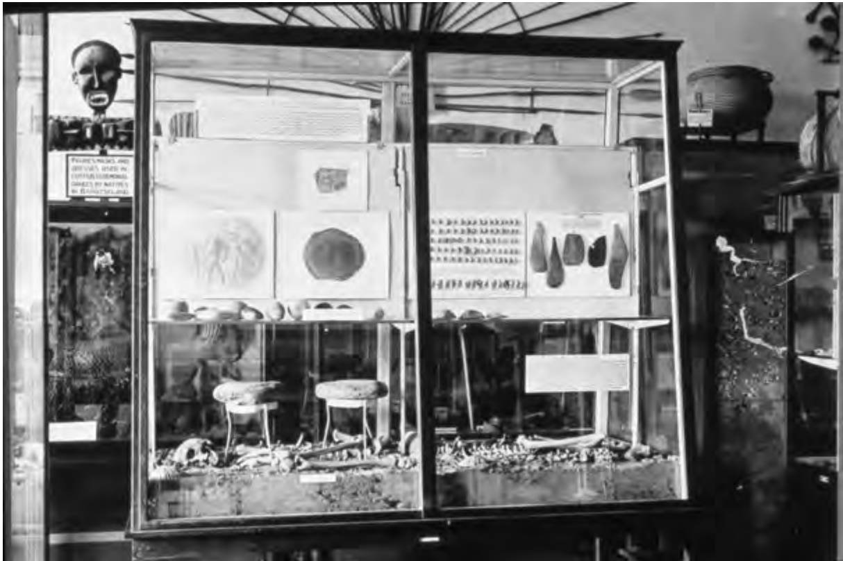
Figure 7. SAM: “Display of stone implements, paintings etc.” at the top of the stairs, 1897.
