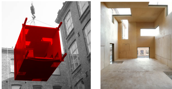
Figure 46: Images showing Rucksack House being lifted by crane during installation (left) and the interior view of the addition (right).
