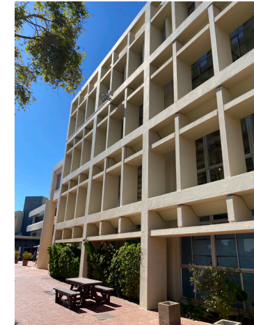
Figure 11: The facade of the campus's student center makes use of a concrete brise soleil that also performs a structural role.
