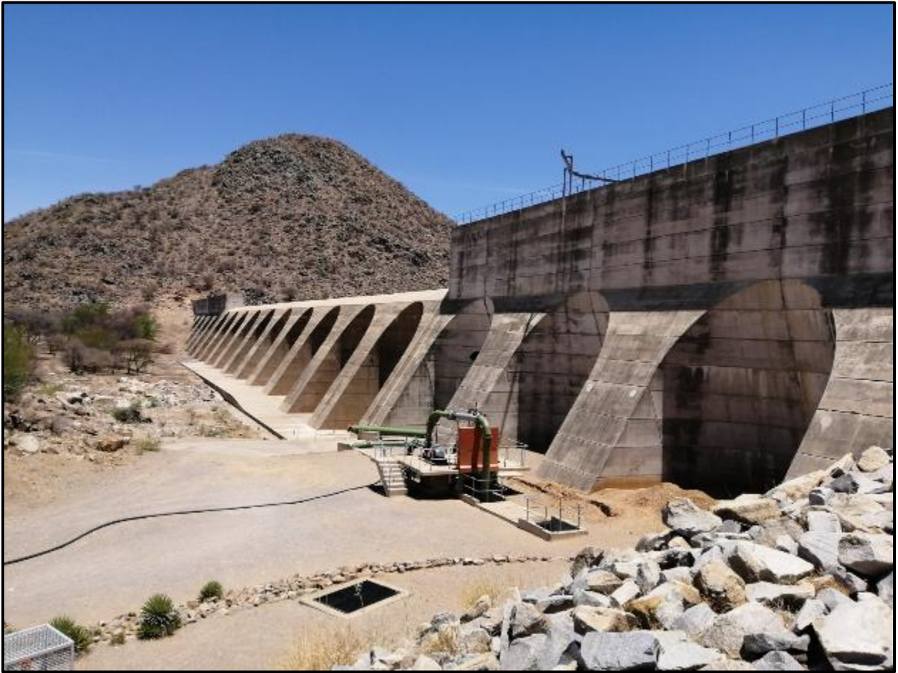
Figure 24: Otjivero Dam Wall
