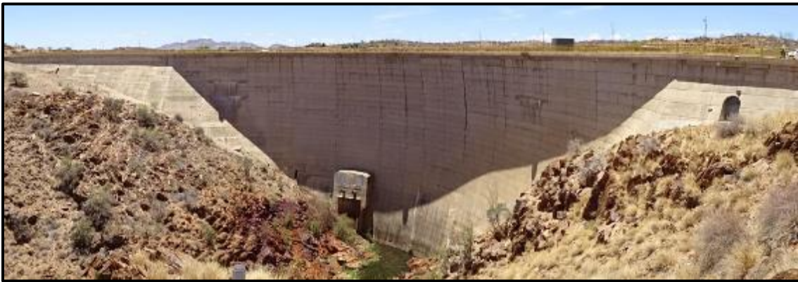
Figure 18: Oanob Dam Main Wall
