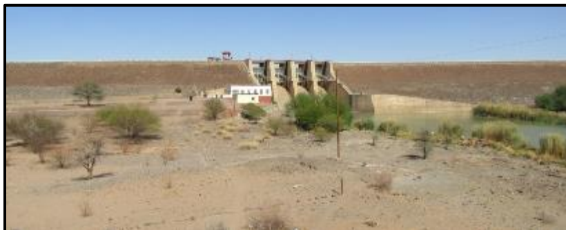
Figure 29: Hardap Dam Spillway and Embankments
