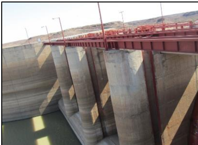
Figure 30: Hardap Dam Upstream of Spillway Section
