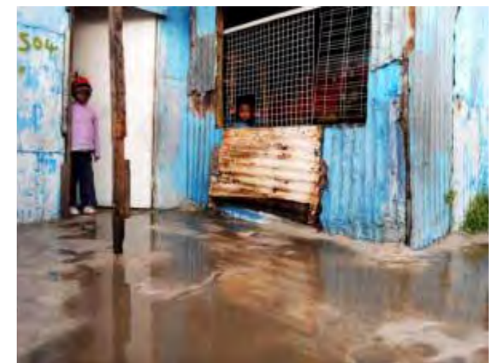
Flooding in Philippi (iol, 2012)
