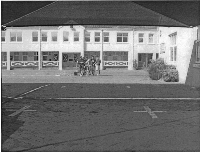
Figure 8.3: View of Building 1 from corner of Building 2
