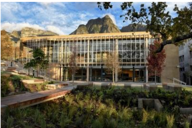
Figure 22 showing East façade of NLT, with grills for growth of creepers
