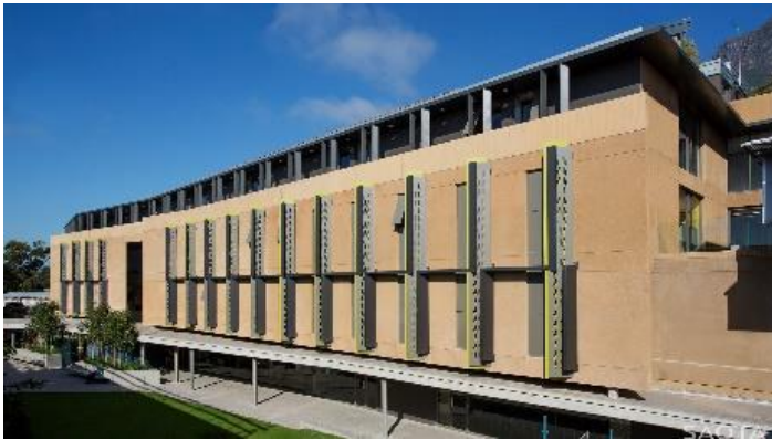
Figure 19 showing East façade of NEB, with vertical grills for shading
