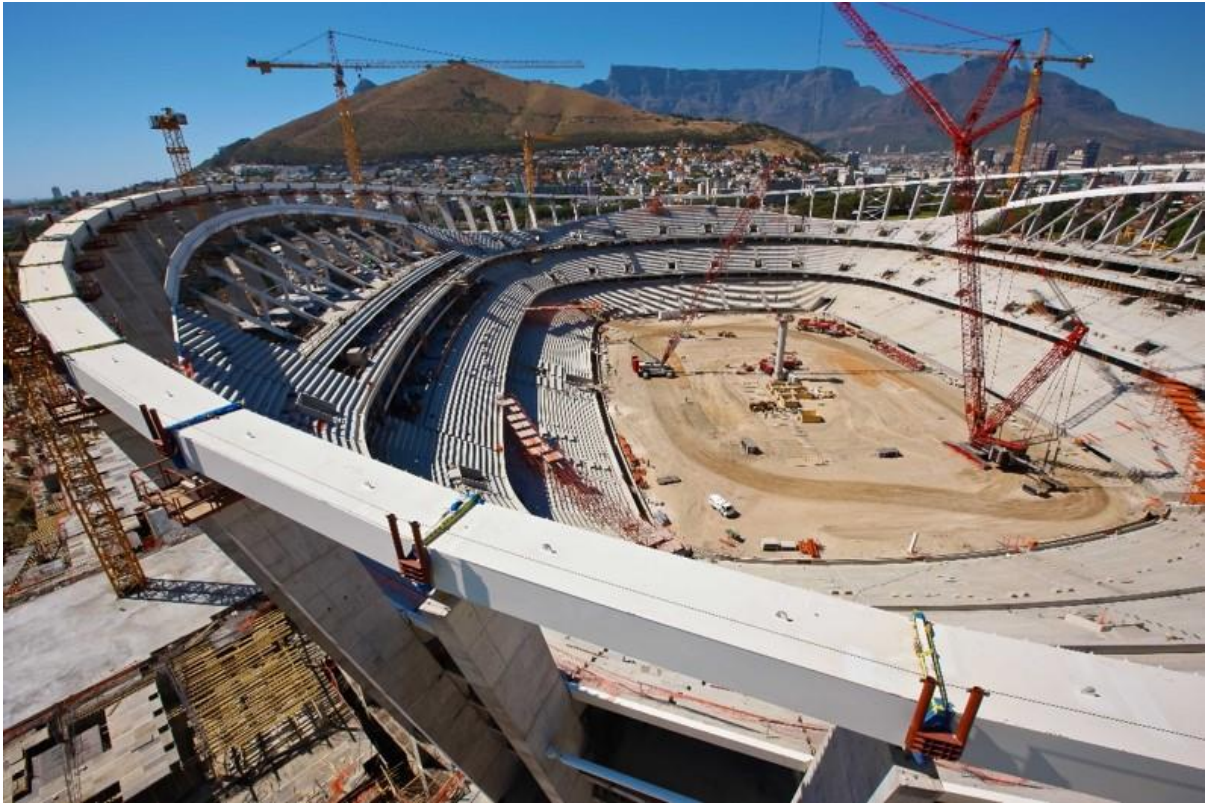
Figure 28: Cape Town Stadium during Construction 1 (Henry Fagan and Partners, 2015)
