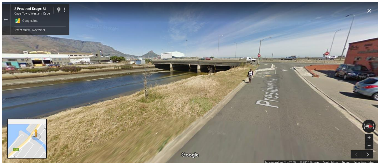
Figure 27: Google Street View of Salt River Bridge (Google Maps, 2018b)
