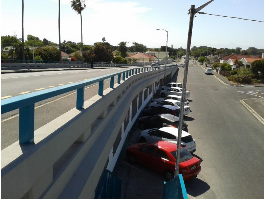
Figure 33: Completed Repairs of Victoria Road Bridge Plumstead. Image taken on 09-11-2016.
