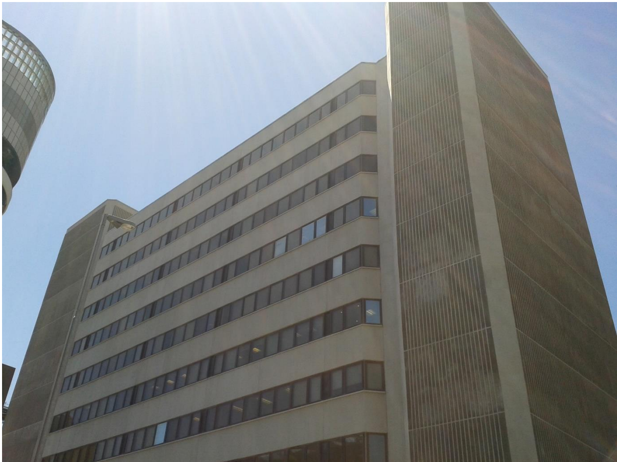
Figure 30: 27 Wale Street View. Image taken on 09-11-2016.
