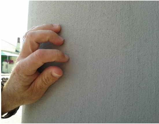
Figure 34: Close-up view of SikaLastic-152 finish. Image taken on 09-11-2016.
