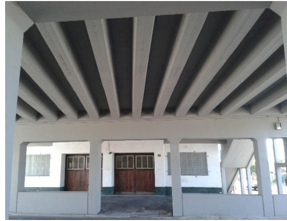
Figure 35: Victoria Road bridge repairs below deck. Image taken on 09-11-2016.
