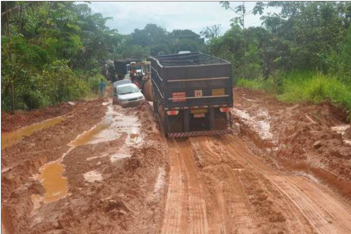
Figure 32: Rutting in unpaved road ( murderiseverywhere.blogspot.com , 2014)
