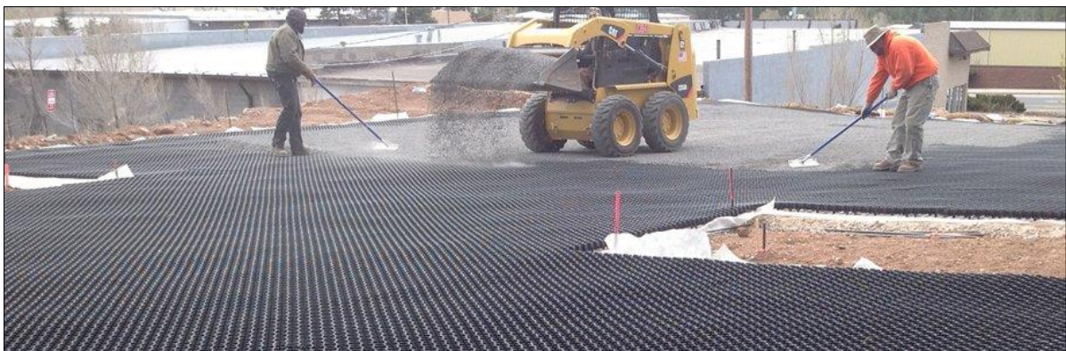
Figure 36: Geosynthetics used in parking lot construction (Typar Geosynthetics)
