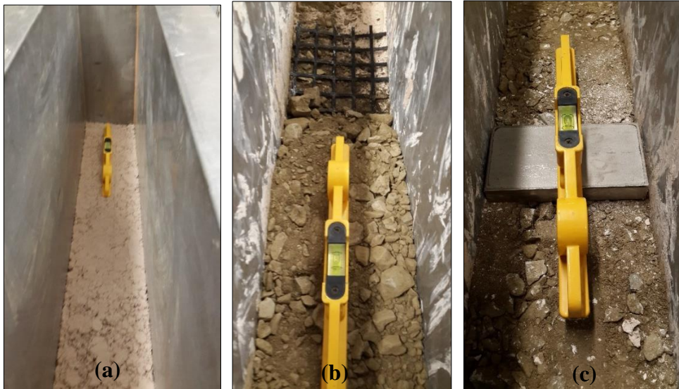
Figure 78: Levelling of the (a) kaolin clay soil, (b) granular material, and (c) model footing (c) during preparation.
