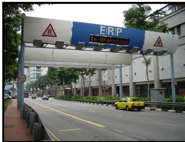
Figure 2.6: Singapore Road Pricing Gantry
