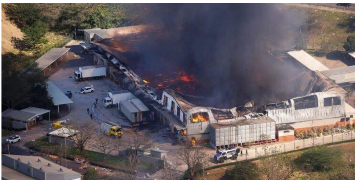
Figure 4.6: Burning warehouse during violence and looting in Durban, July 2021 Uprisings
