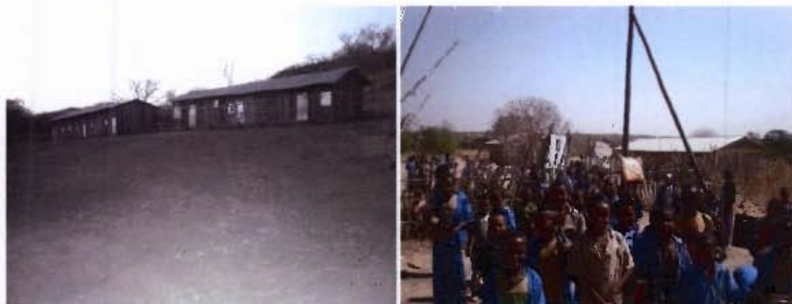
Picture 5: School conditions (the left side is Wodi-Gemzu and the right Das-Gundo)
