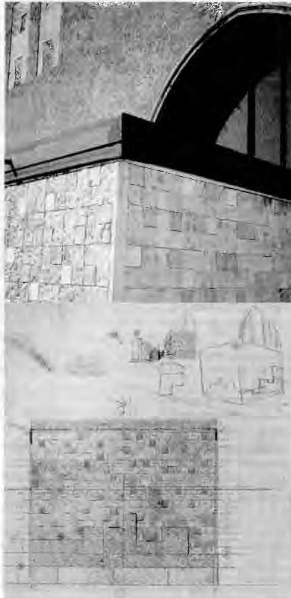
Figure 4: The rough and smooth textures of the local stone on the exterior wall of the gallery extension. Note in the background how existing window openings have been closed off.
