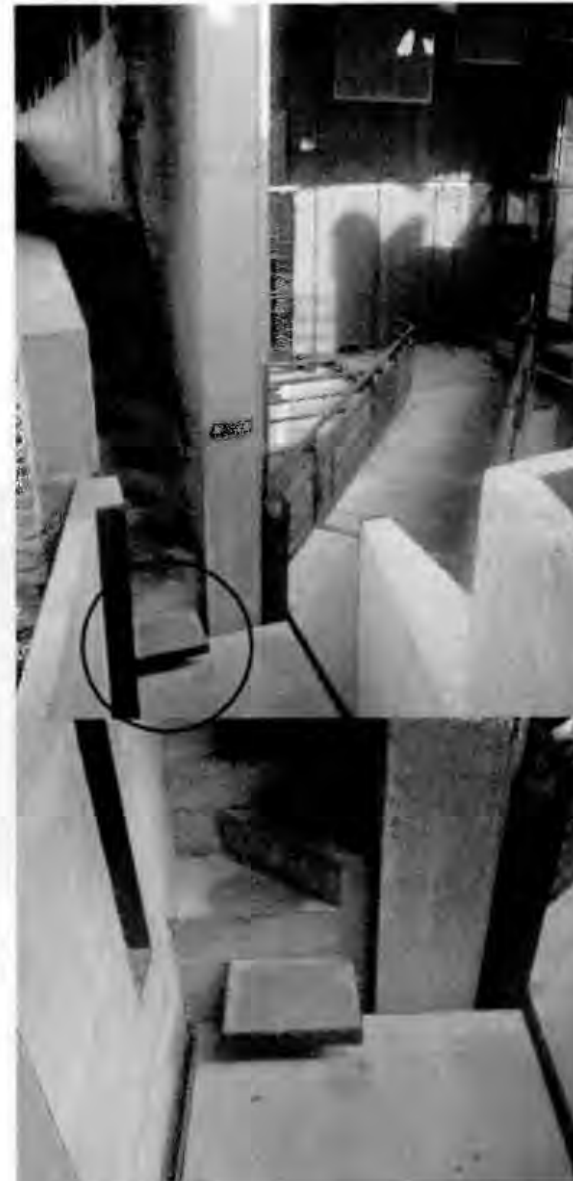
Figure 6: A special gesture is made of the first step of the concrete staircase in the Cangrand space, it acts as a threshold between two different spaces.
