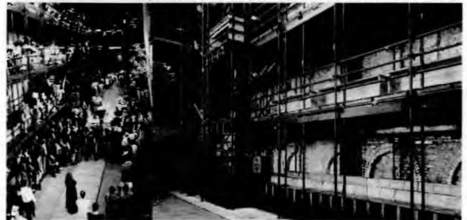
Figure 31: The interior of the theatre during rehearsal.
