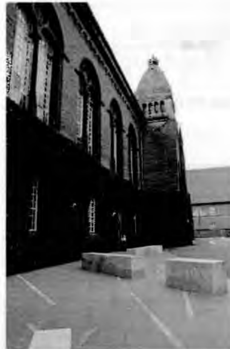
Figure 25: View of the Northwest façade from the North. The entrance is part of the brick Royal Library.
