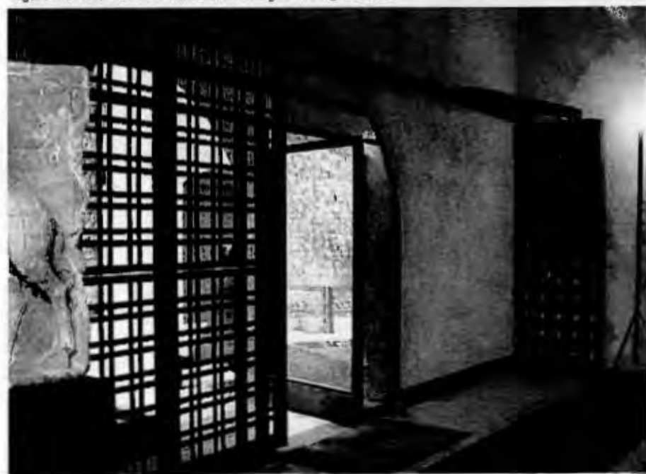
Figure 14: The exit door with steel sliding & folding screen.
