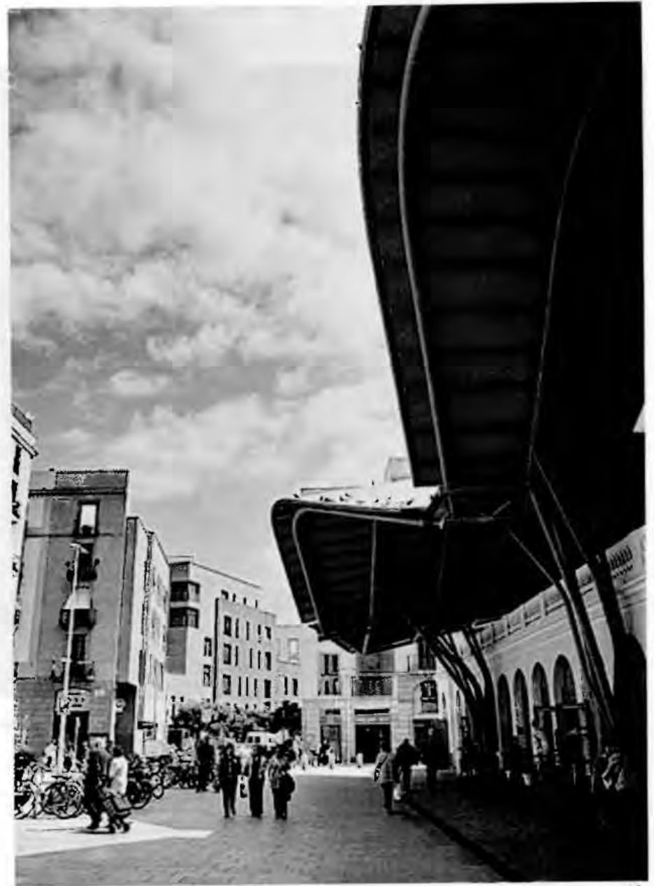
Figure 20: The Santa Caterina Market in Barcelona with its new roof extending over the original walls of the old market building.
