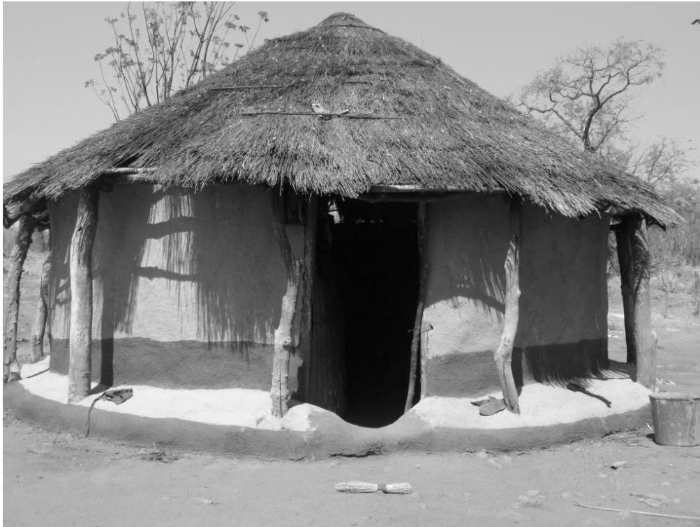
Figure 4.6: Pole and dagga traditional house in a village adjacent to Sikumi. Source: Field picture
