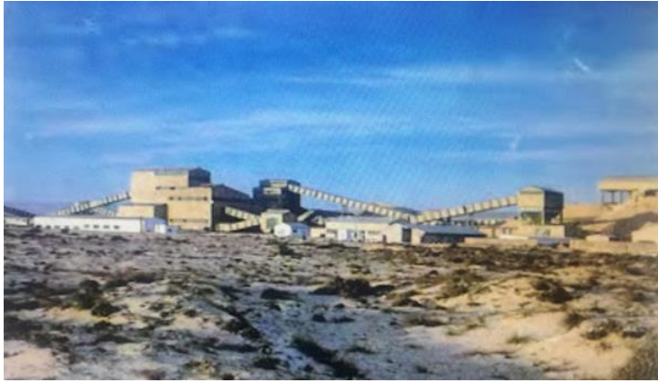
Figure 21 Gravel processing plant at Kleinzee Mine
