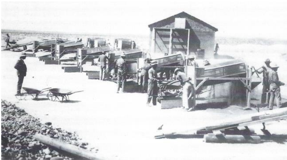
Figure 26 State Alluvial Diggers putting gravel through trommel sieves (classifiers) during the early 1930s. Under the watchful eye of the overseer (nickname "The Pole", left). (Pieter Coetzer, Baai van Diamante, 1997)
