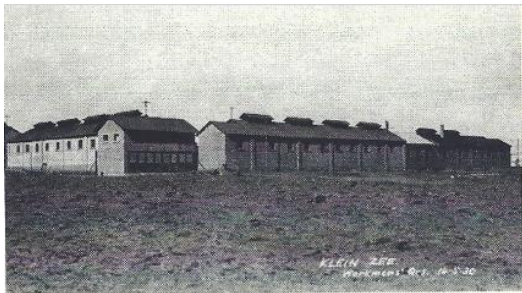
Workers' Quarters (Compound)
