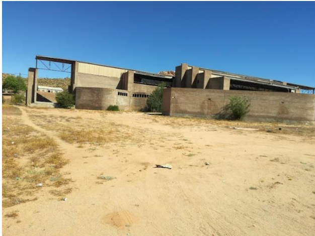
Figure 44 Award-winning multi-purpose hall donated to the community of Steinkopf by De Beers Namaqualand Mines. Abandoned today. (Own Collection)
