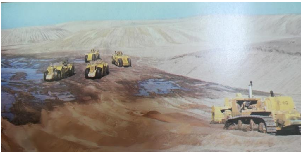
Figure 20 Giant scrapers and bulldozers removing the sand overburden.
