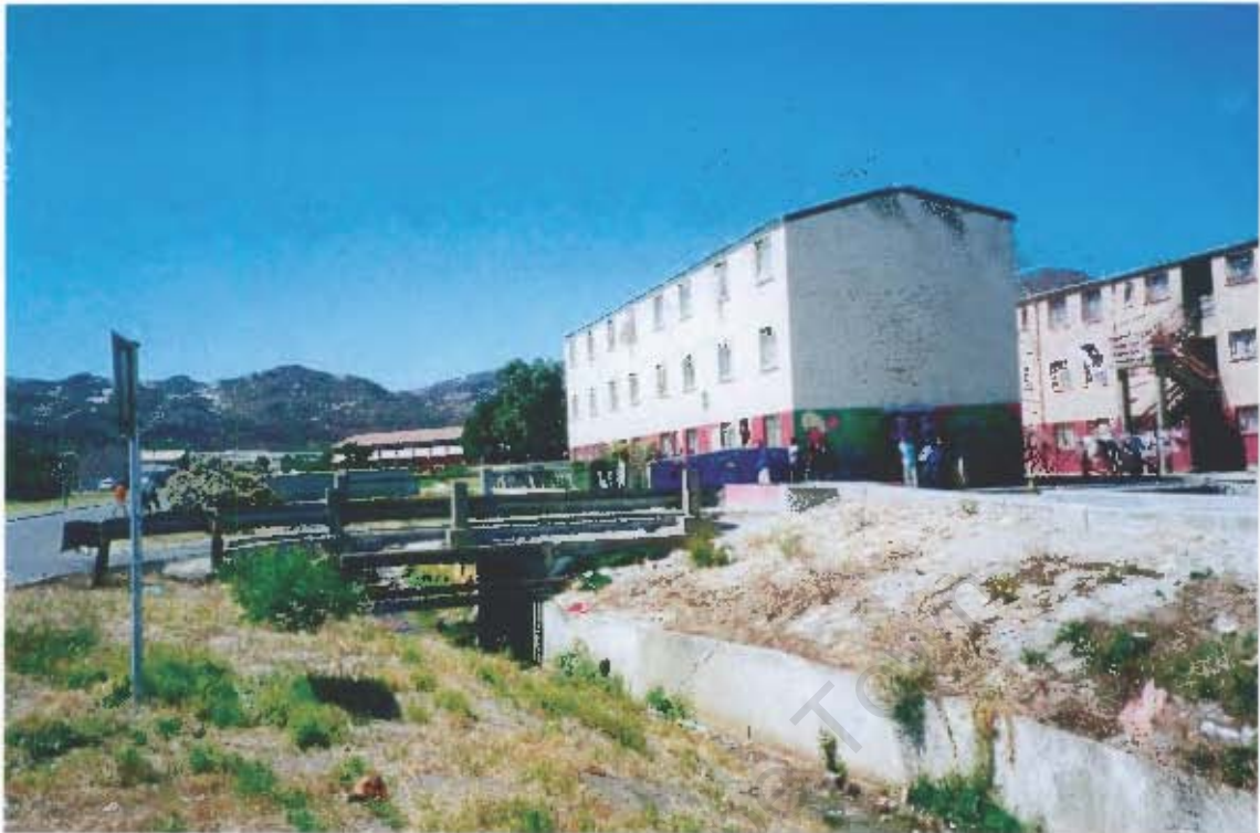
Figure 3-4 : Hostels and a section of the canal draining Ocean View
