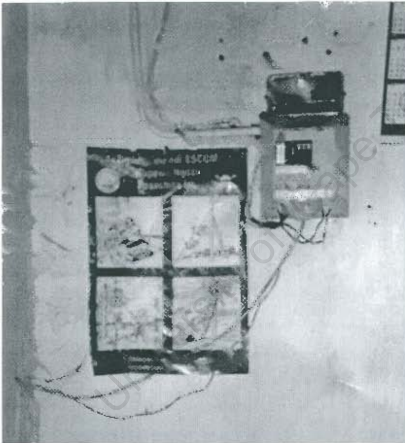
Picture 2: A compact ready board with some of wires inserted directly into sockets
