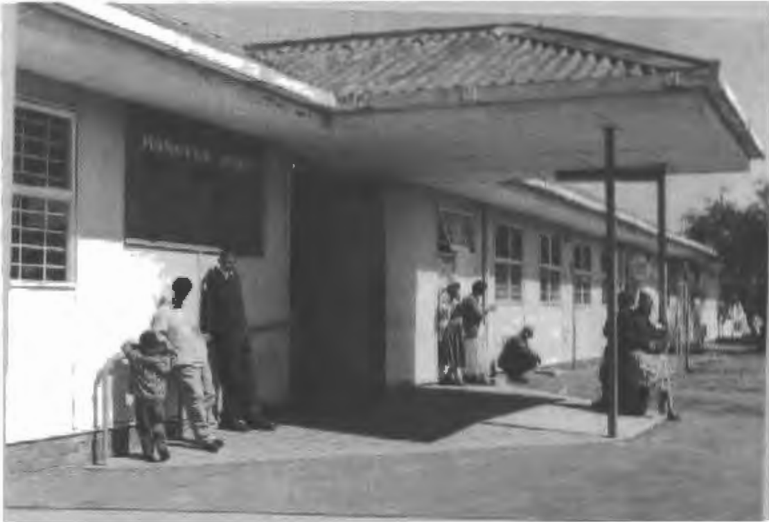
Figure 1.1 The Main entrance to Hanover Park CHC
