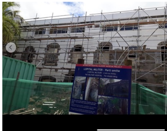
Figure 25: The Building under renovation
