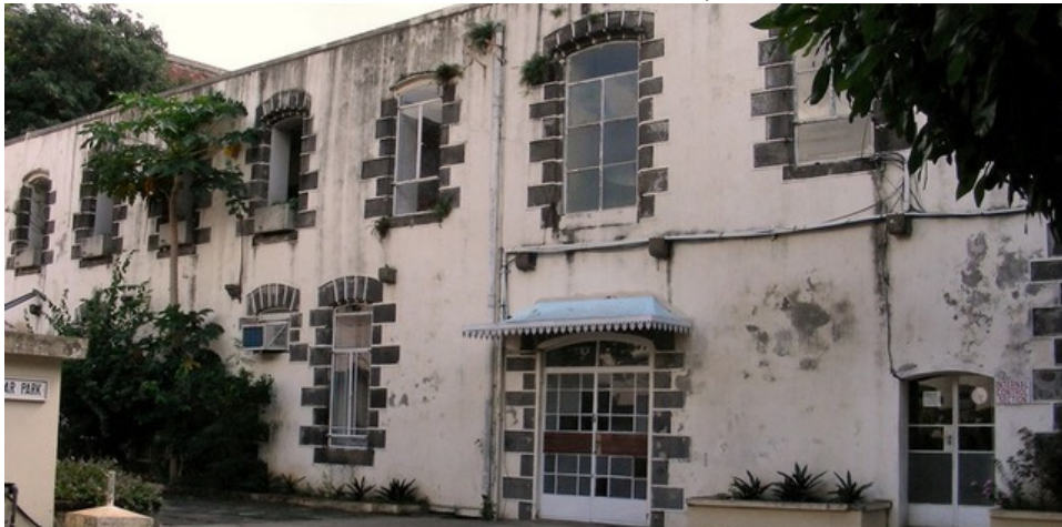
Figure 21: The hospital as government administration buildings with ad-hoc upgrades, prior to renovation. The local basalt rock window surround details are clear in this image. Photograph, Le Mauricien (2020)
