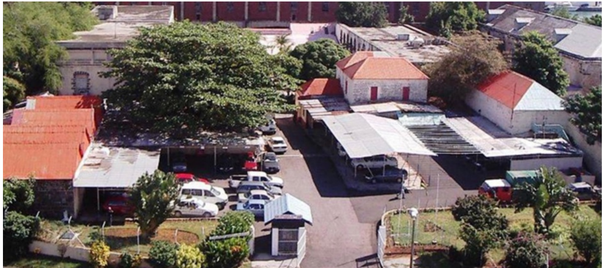
Figure 23: A Modern Aerial View of the Complex showing the accumulation of ad-hoc additions of carports and storage facilities.(Le Mauricien, 2020).
