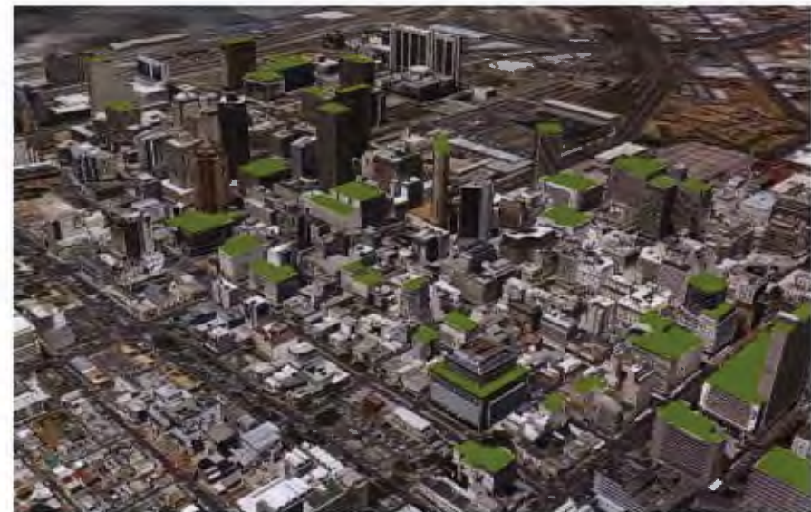
The picture shows the potential for roof space utilization in the Cape Town CBD area.
