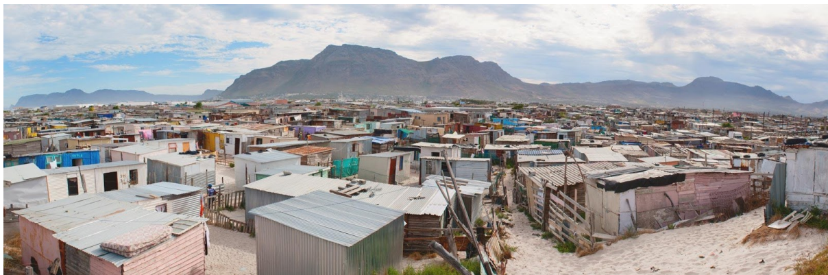
Figure 5.3: Example of residential structures of Vrygrond Community (Google Maps, 2017)
