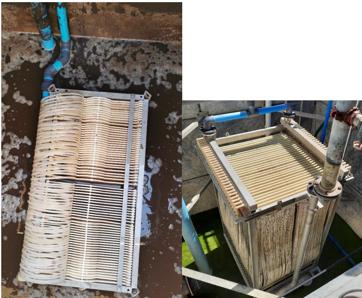
Figure 7: Pictures of flatsheet (left) and hollow fibre (right) membranes used in industry.
